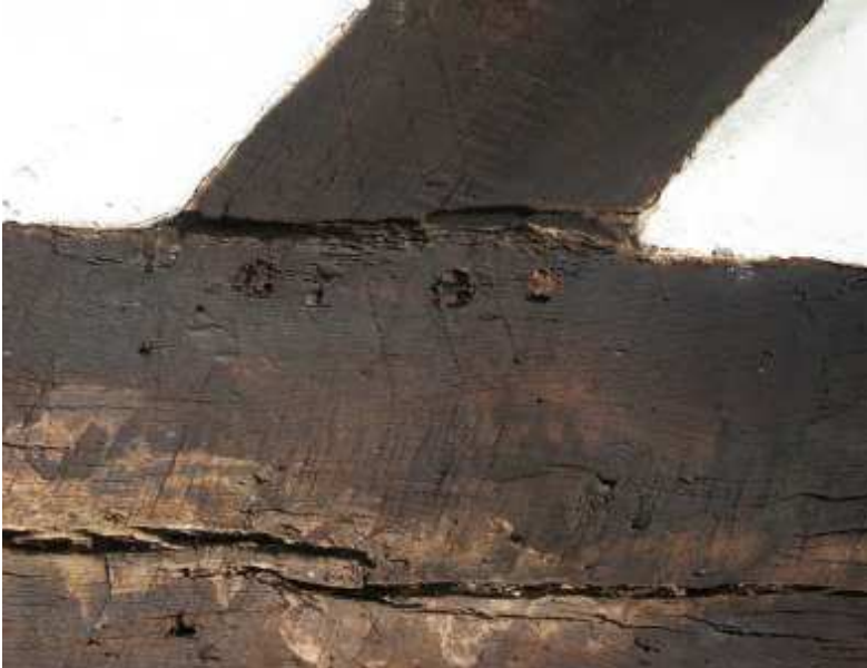
wing truss 4: carpenter's marks on tie-beam and strut
