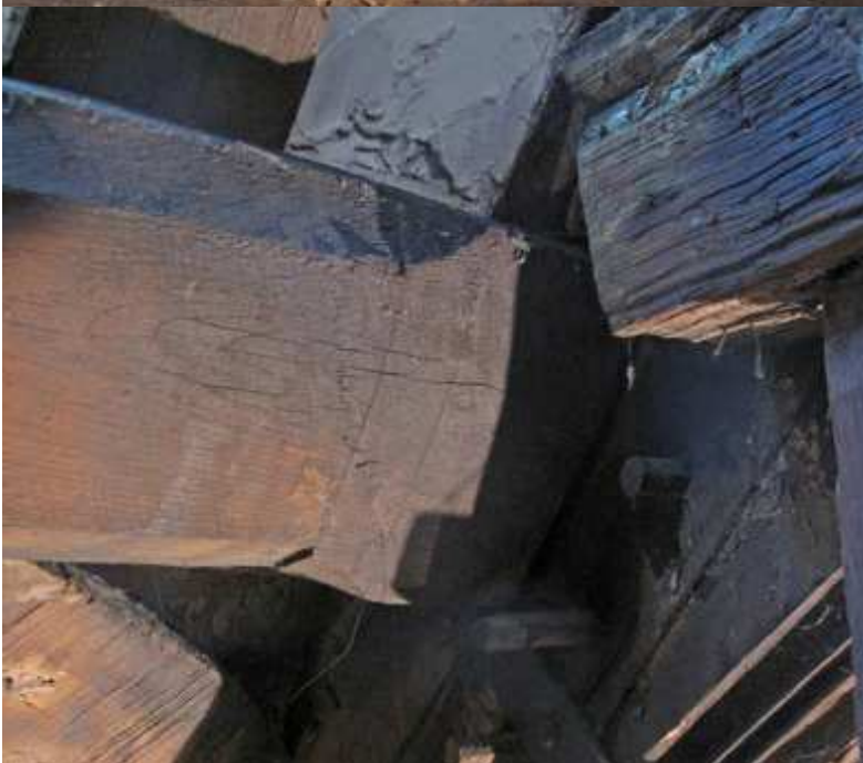
chamfered purlin at truss 3: carpenter's marks
