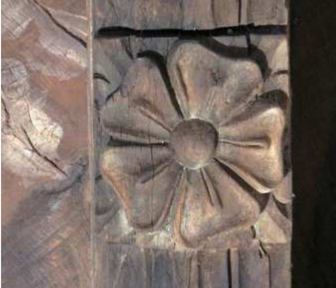
Truss 2: west rose
