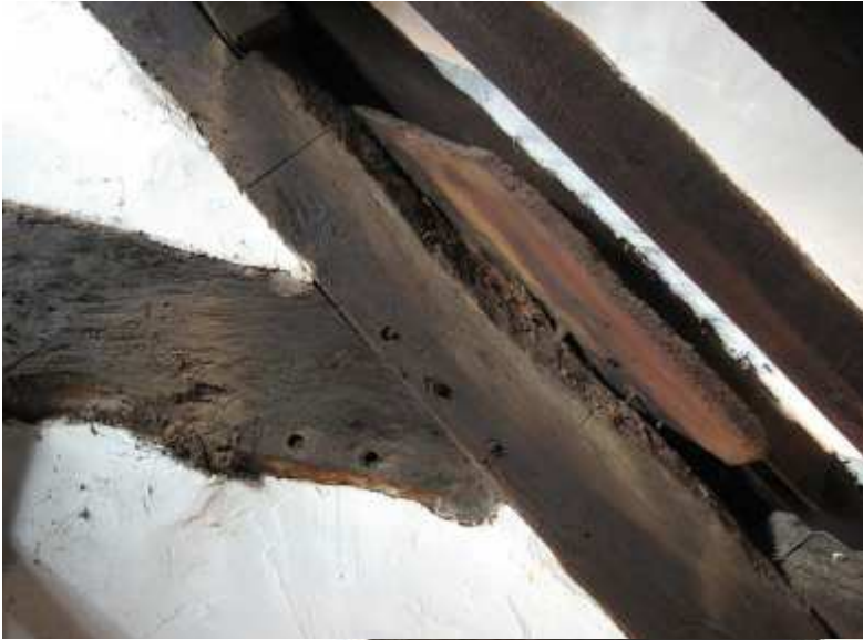
Truss 4: carpenter's marks on principal
