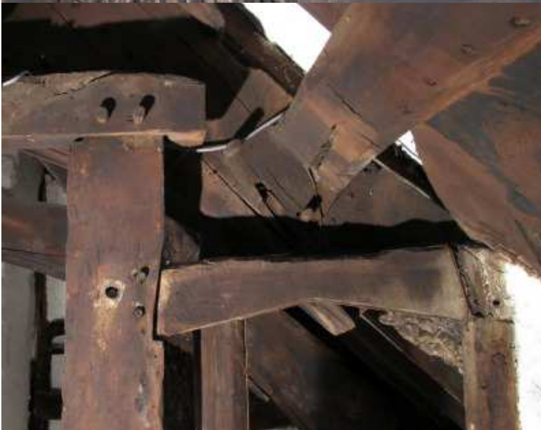
first floor partition; false four-centred door head and carpentry
