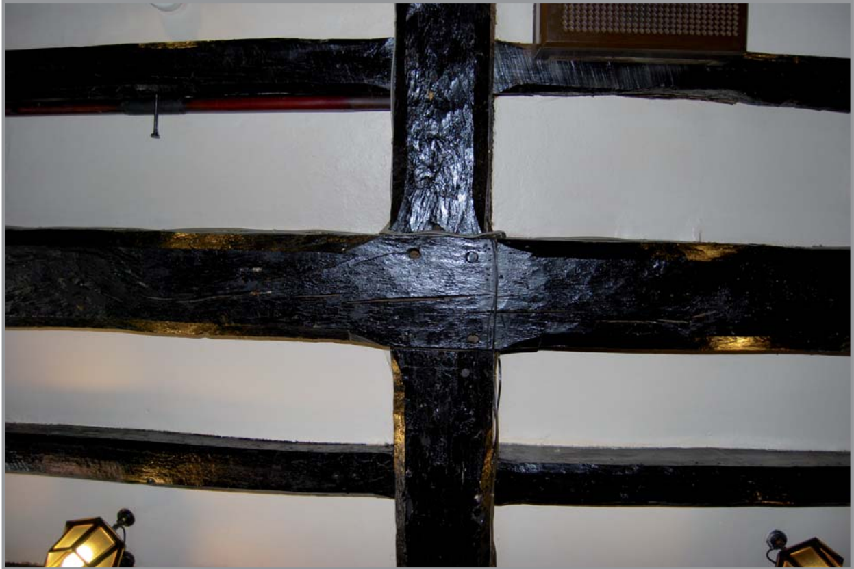
Plate 11: Image showing axial beam and transverse beam
