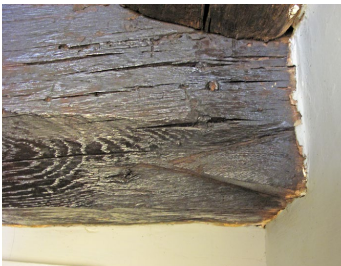
Large beam on the north side of the passage with broad chamfer and broach stop at east end
