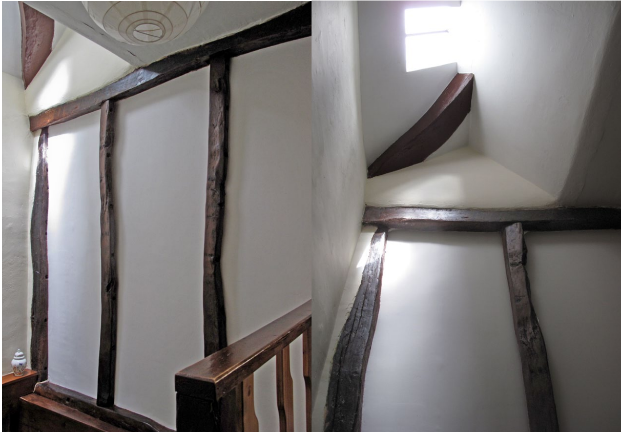
stud and rail partition with holes for staves, wattle and plaster
