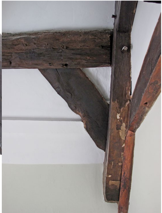
Collar-beam truss, principal, purlin and wind brace joints
