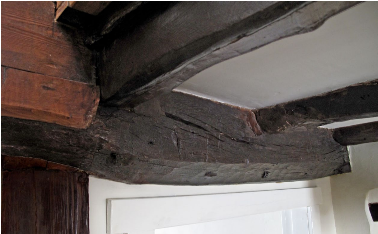
Large beam on the north side of the passage with broad chamfer and broach stop at east end
