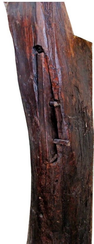
wall-post with mortice, tenoned and pegged joint
