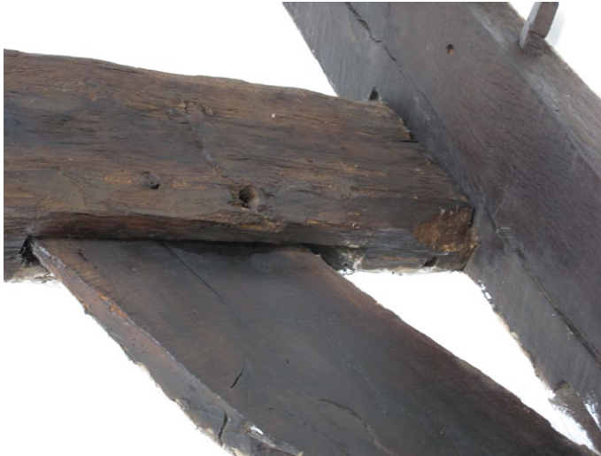
Collar-beam truss, principal, purlin and wind brace joints
