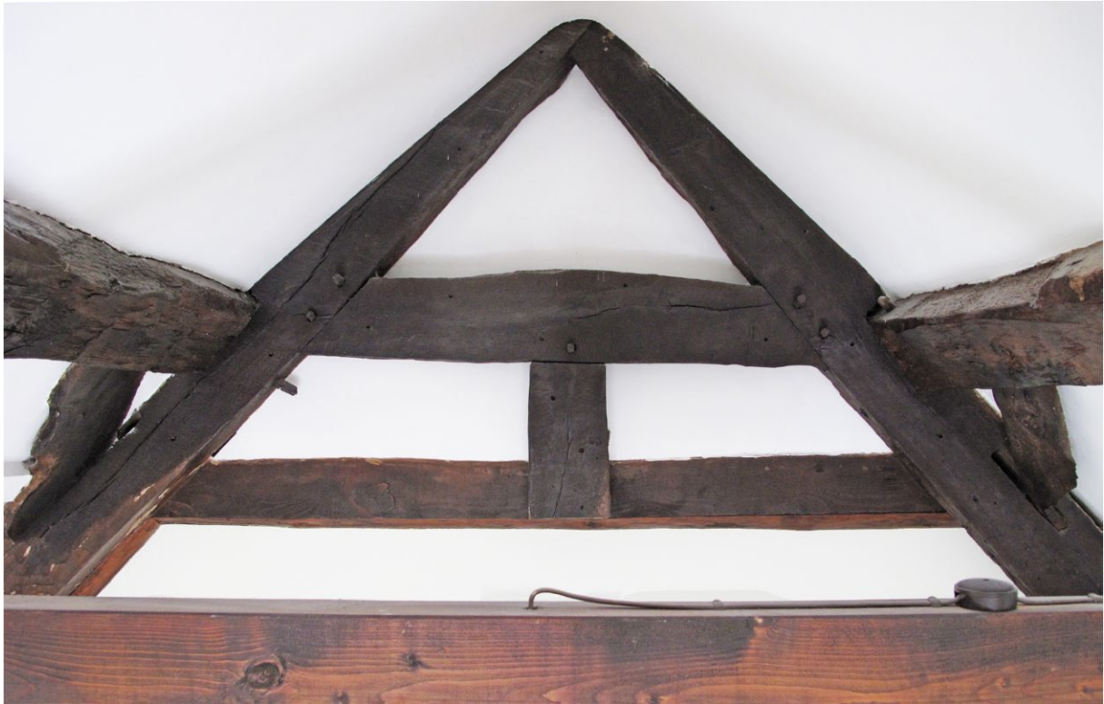
Collar-beam truss against the north wall of the south upper room. The near, square beam is modern and nothing to do with the truss. The lower of the two collars is a secondary feature, fixed behind the principals. A tie-beam has been cut away and the crown post, down from the original collar, has been truncated
