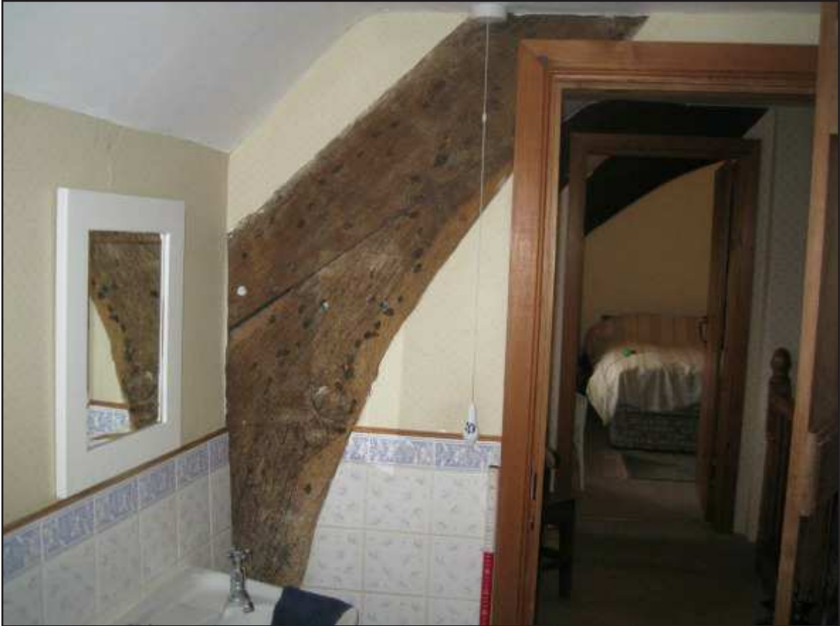
Plate 11: The eastern side of the northern face of the northern cruck which forms the northside of the screens passage; view from the north.
