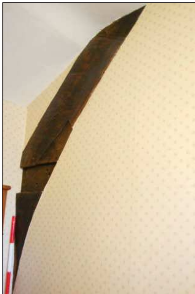
Plate 10: The eastern side of the southern face of the northern cruck which forms the southside of the screens passage
