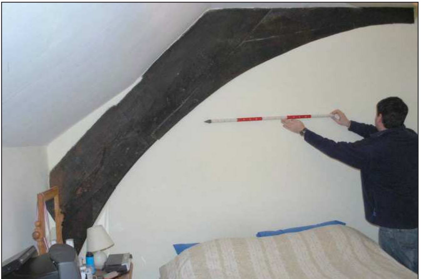
Plate 6: The eastern side of the northern face of the southern cruck which divides the hall; view from the north.
