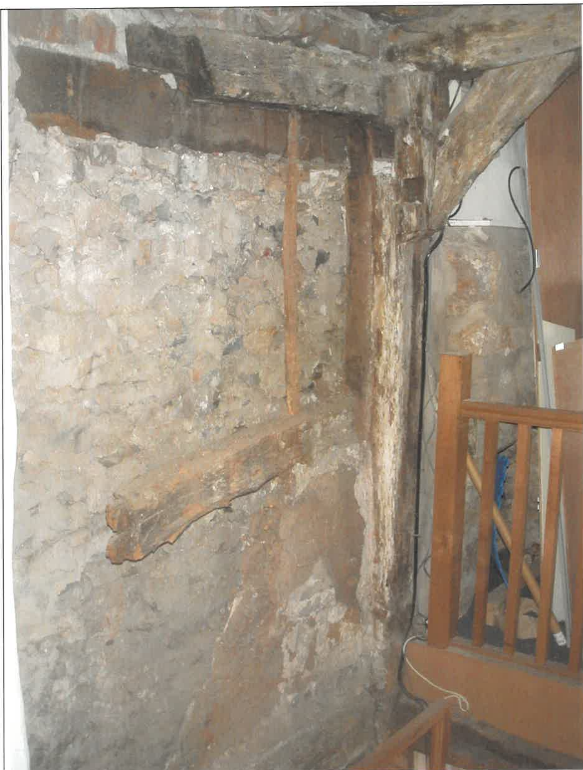
Plate 7 Oak framed wall on north side (with wattle & daub infill)
