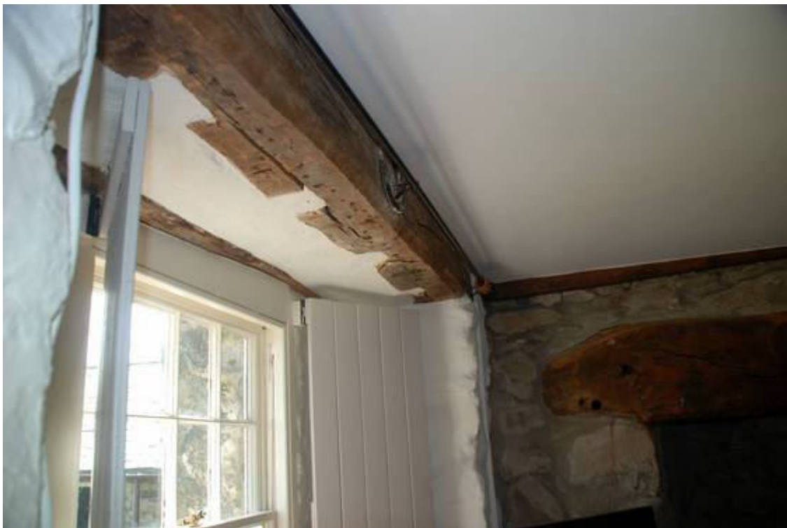
Plate 12: Re-used tie beam
