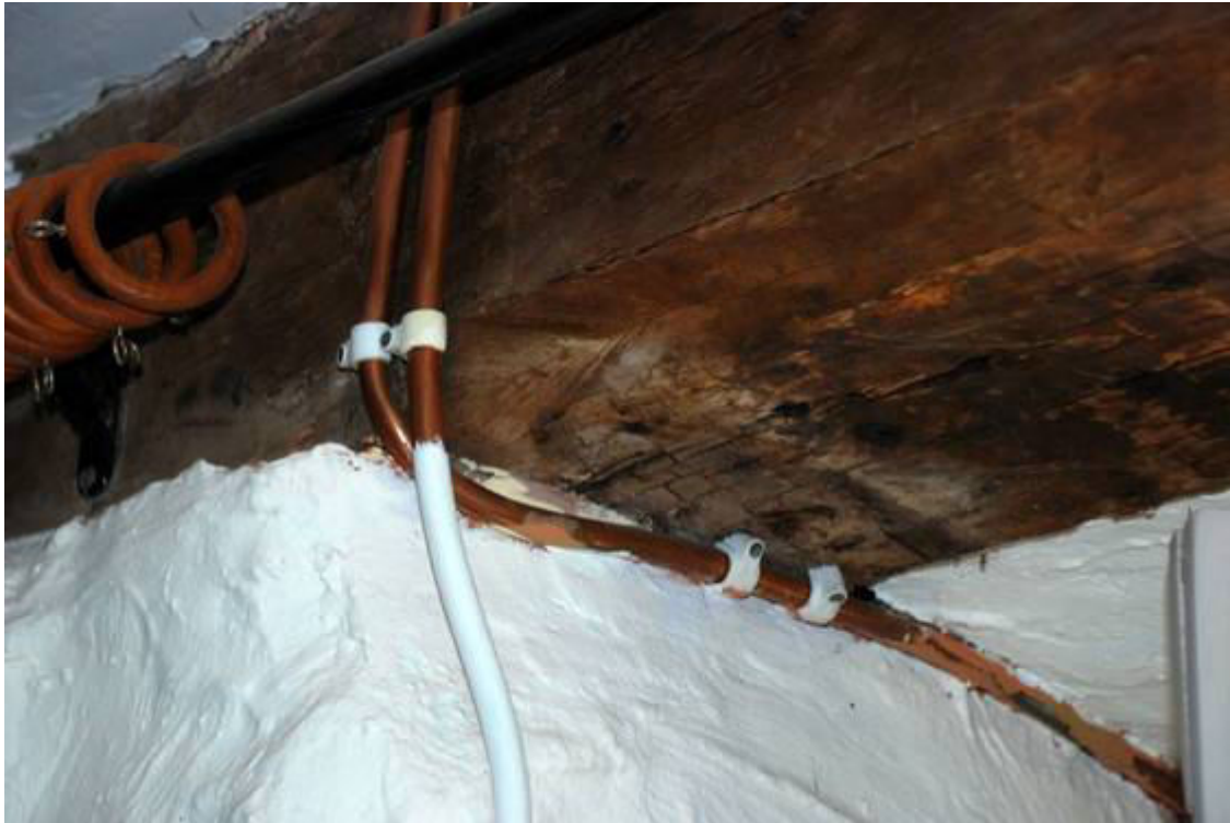
Plate 11: Broach stop and chamfer on re-used tie beam
