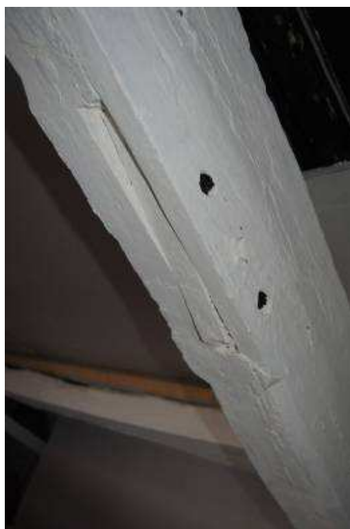
Plate 27: Truss T2; sawn off primary collar
