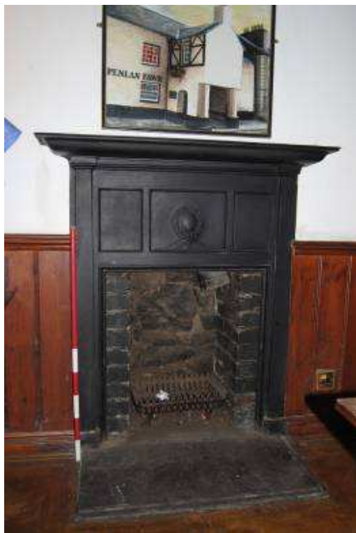
Plate 11: Inserted FP, east wall.
