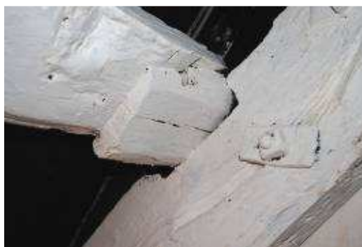
Plate 29: Detail of purlin scarf
