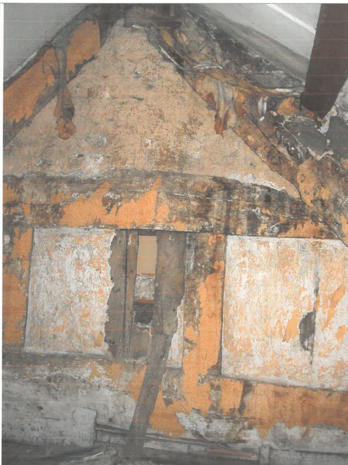
Plate 6 attic floor of No.16a, truss in north wall (centre)
