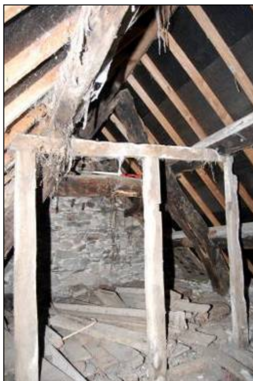
Plate 21: Joints in top of lateral beam
