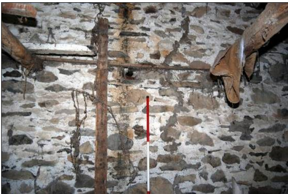
Plate 20: Lateral beams and socket for missing support
