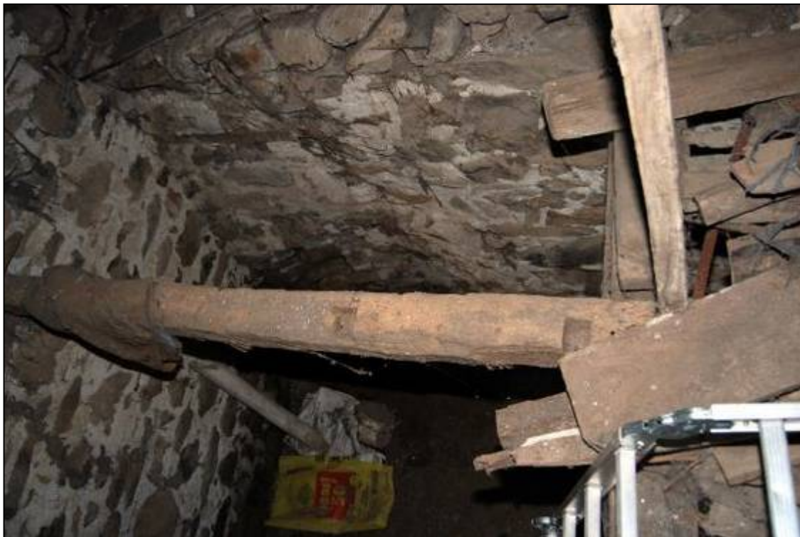
Plate 21: Joints in top of lateral beam
