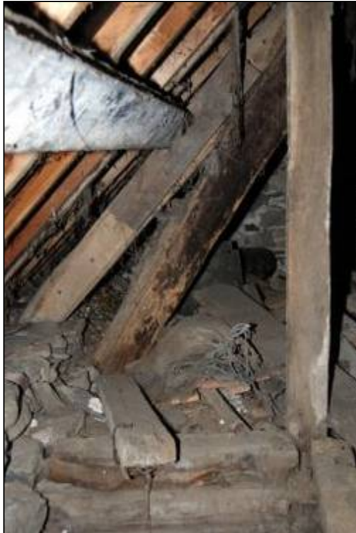
Plate 26: Detail of southern blade of Truss 1
