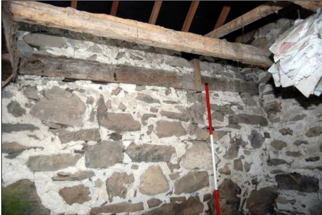
Plate 18: Rail in north wall
