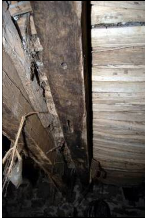
Plate 17: Evidence for the partition below Beam 4
