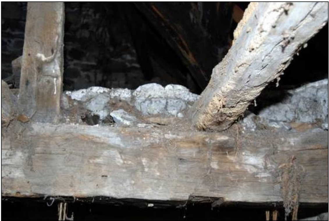
Plate 16: Plaster surface of the platform
