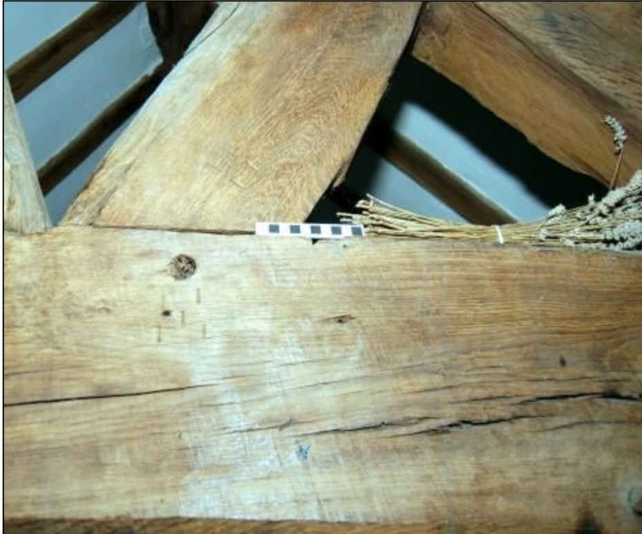
Plate 52: Carpenter's marks on Truss 2.
