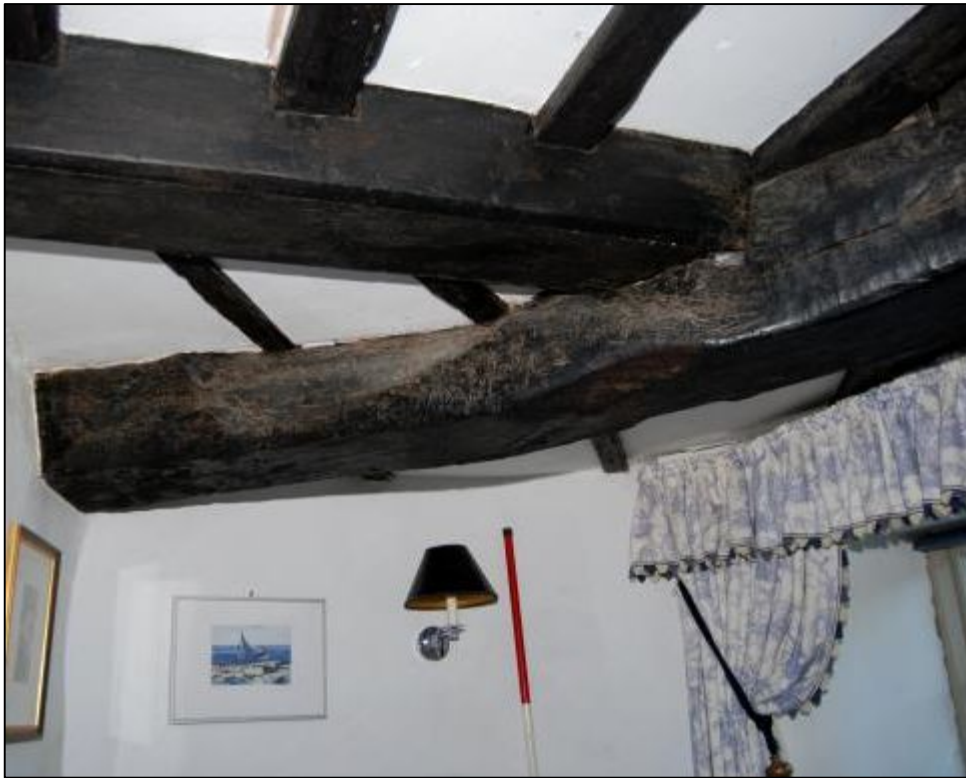
Plate 27: Arrangement of the beams in the bathroom
