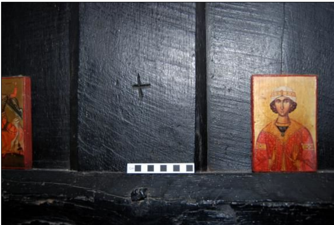
Plate 19: Carpenter's mark on the ground floor partition
