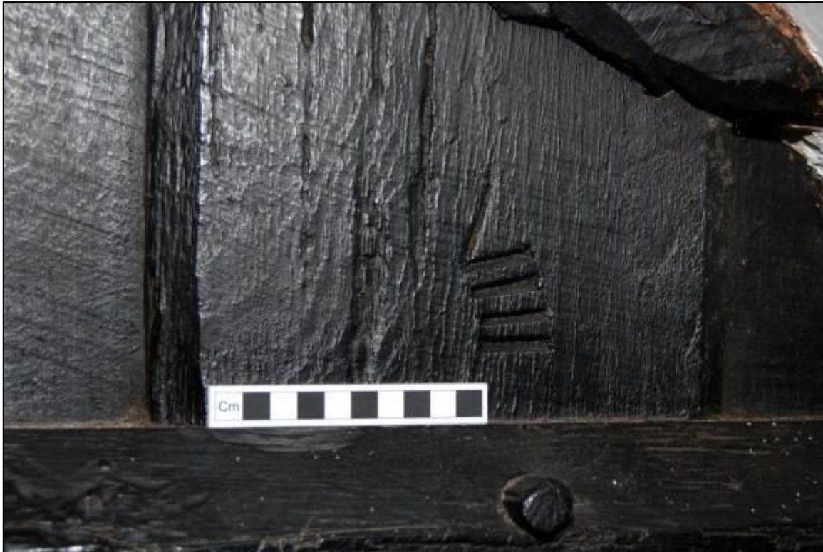
Plate 18: Carpenter's mark on the ground floor partition
