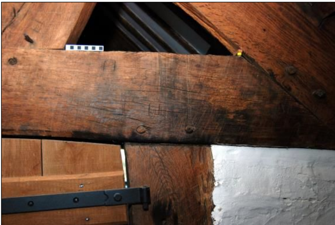
Plate 50: Carpenter's marks on Truss 1
