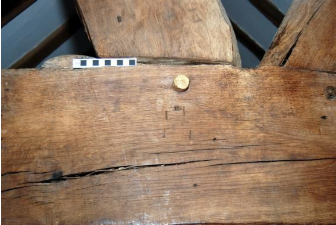
Plate 51: Carpenter's marks on Truss 2
