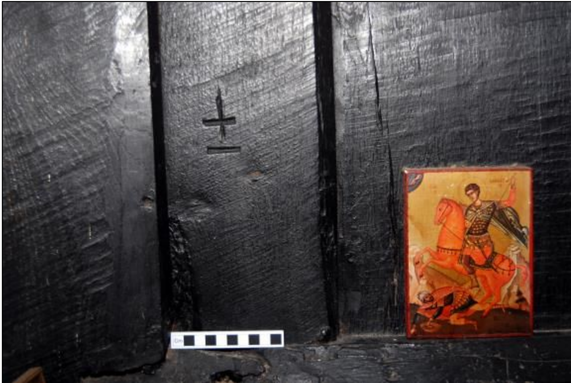
Plate 20: Carpenter's mark on the ground floor partition
