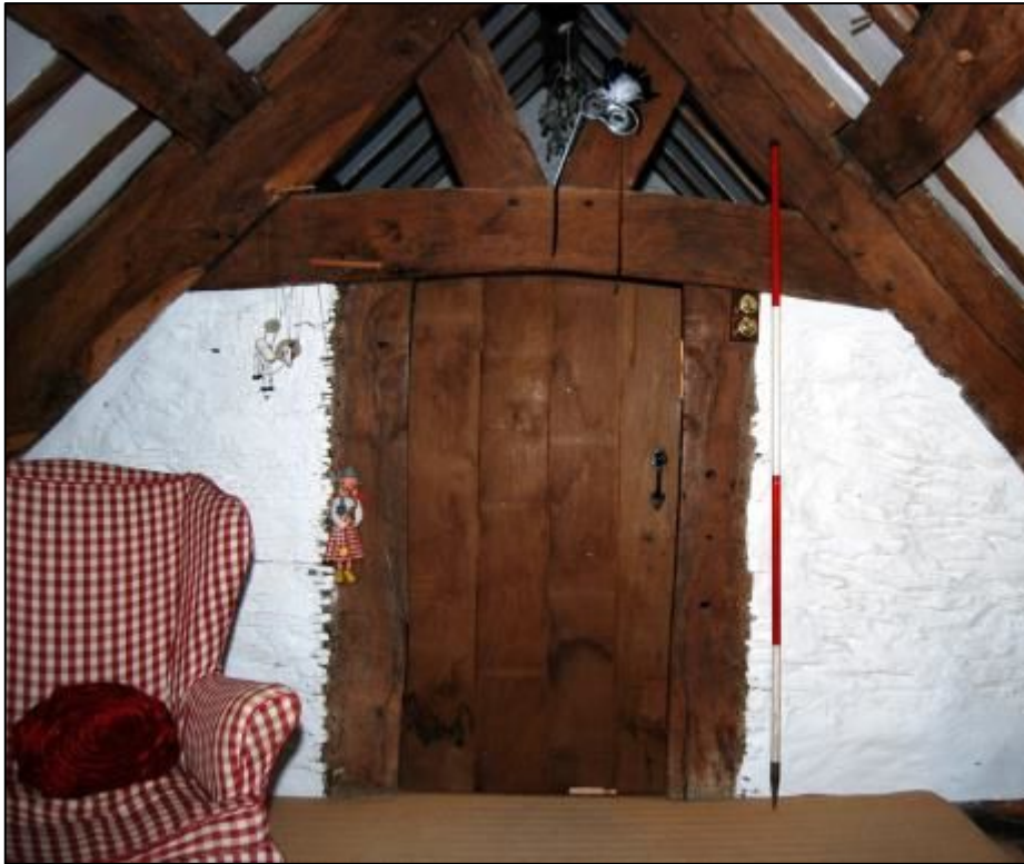
Plate 42: Wattle and daub partition below Truss 1
