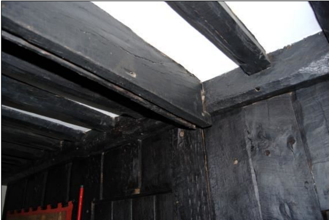
Plate 24: Slot below a joist in the parlour
