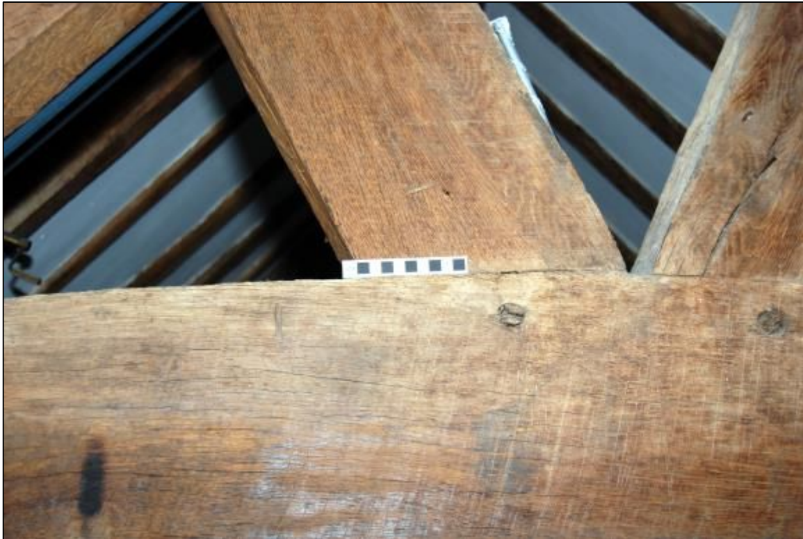
Plate 49: Carpenter's marks on Truss 1
