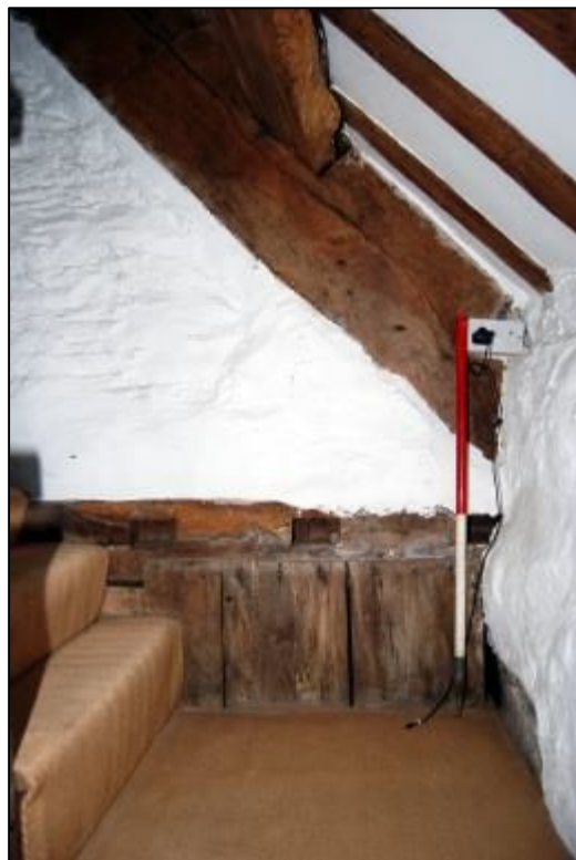
Plate 43: Post and panel partition in the stairwell below Truss 1
