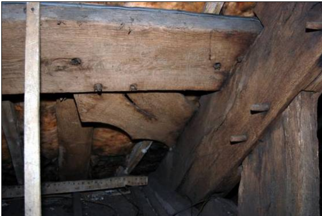
Plate 47: Upper, northern windbrace associated with Truss 1
