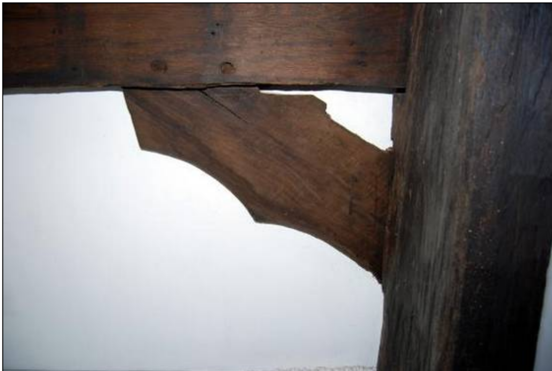
Plate 41: The northern windbrace at the eastern end of Truss 3
