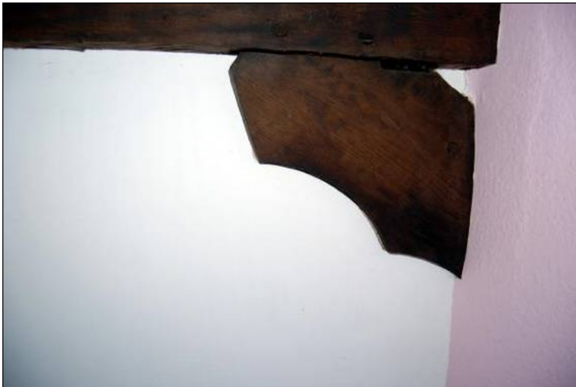
Plate 38: Cusped windbrace for Truss 2 in northern bedroom
