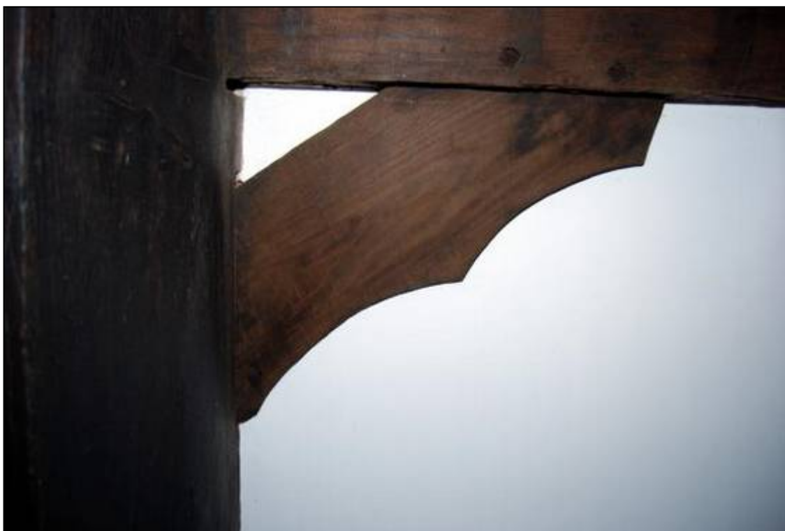
Plate 42: The southern windbrace at the eastern end of Truss 3
