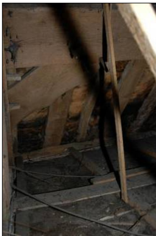
Plate 48: Upper southern windbrace associated with Truss 1
