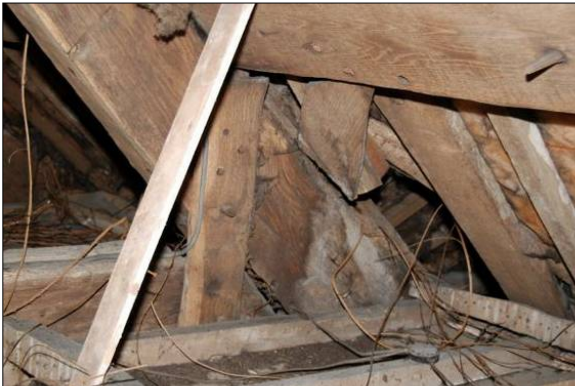
Plate 53: Upper southern windbrace associated with Truss 2
