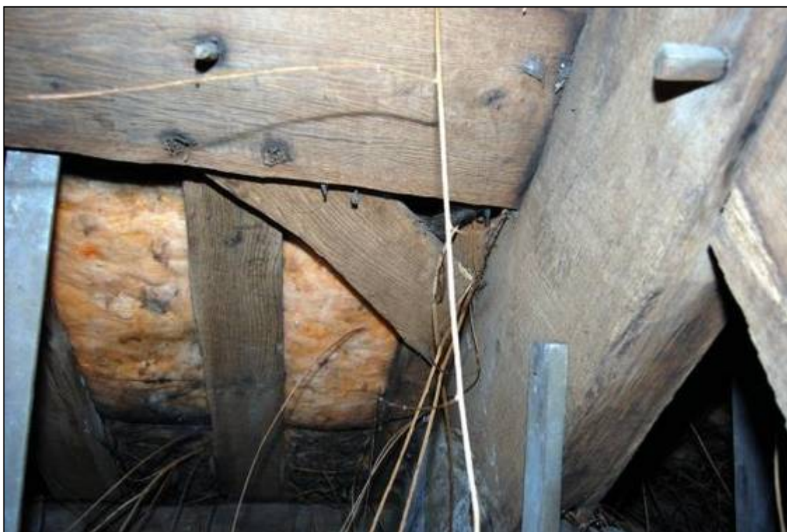
Plate 58: Upper northern windbrace on the western side, associated with Truss 3
