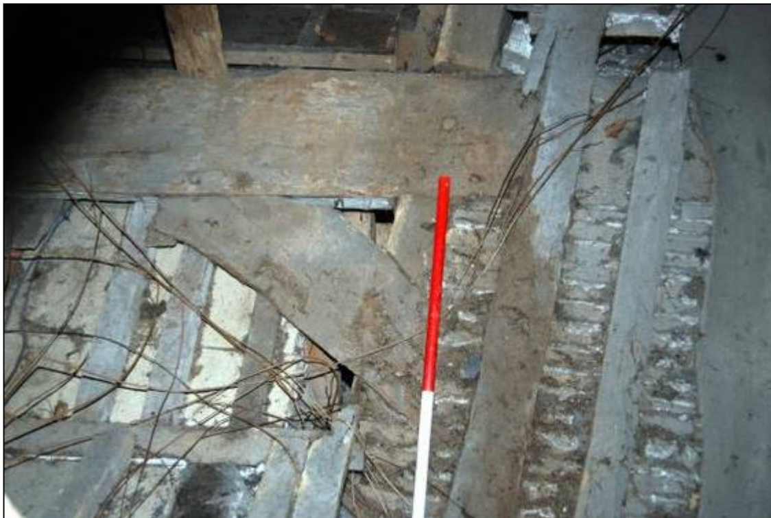
Plate 49: The lower, northern windbrace associated with Truss 1
