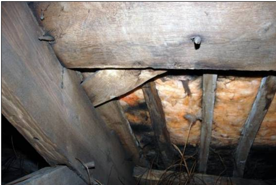
Plate 55: Upper, northern windbrace on western side, associated with Truss 2
