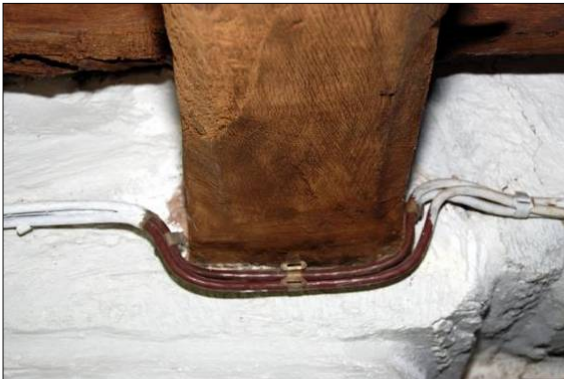
Plate 13: Chamfering and stop on the central beam in the porch
