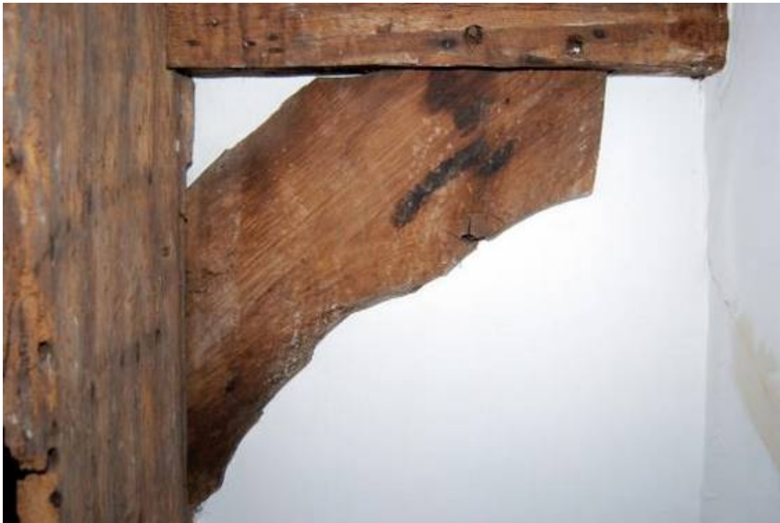
Plate 36: Windbrace in corridor at eastern end of Truss 2
