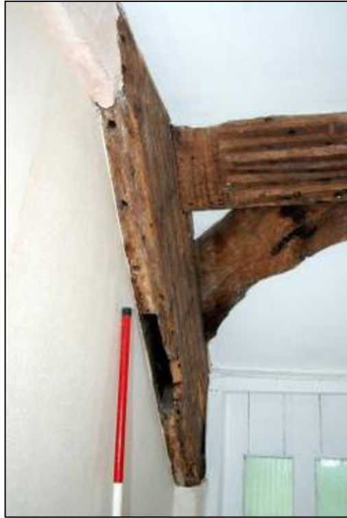
Plate 37: Socket for the tie beam at the eastern end of Truss 2
