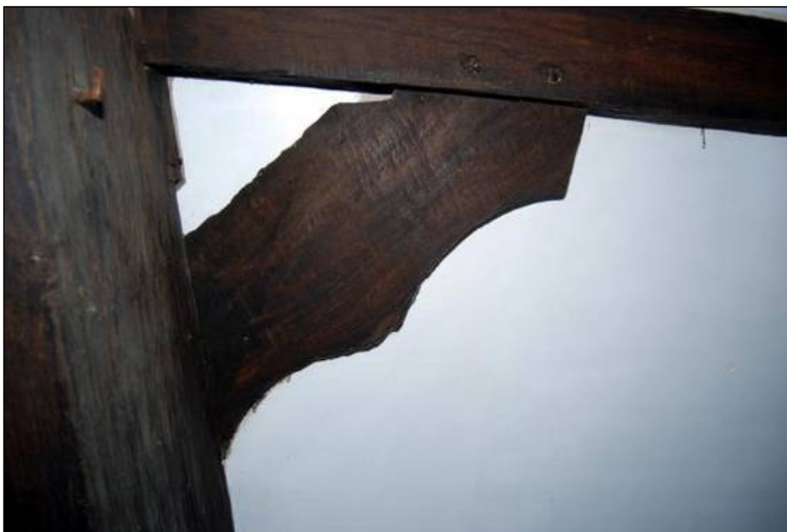
Plate 44: The northern windbrace at the western end of Truss 3
