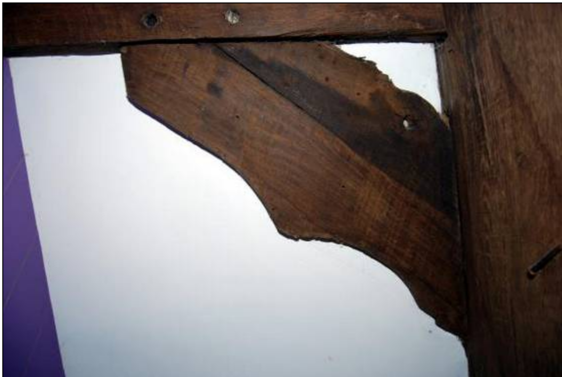
Plate 43: The southern windbrace at the western end of Truss 3
