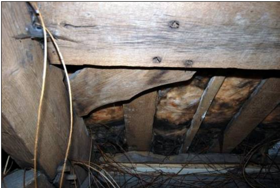
Plate 57: Upper, southern windbrace on the eastern side, associated with Truss 3
