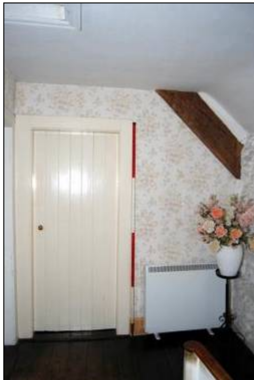
Plate 28: Base of Truss 5, exposed on the landing
