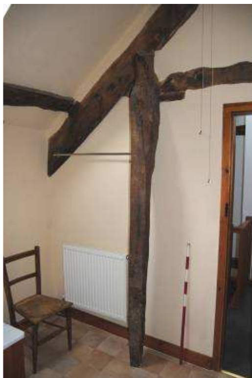
Plate 19: Inserted strut to T2 [1F03].
