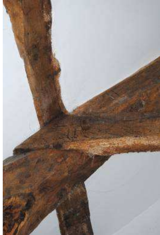
Plate 16: Detail of lap jointing and square pegs; NB: carpenter's numbering ('11') to collar and principal.
