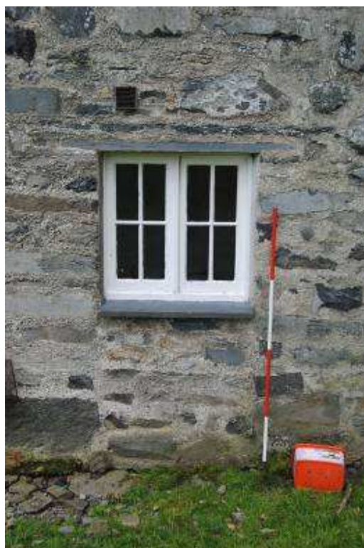
Plate 5: North elevation; door converted to window.
