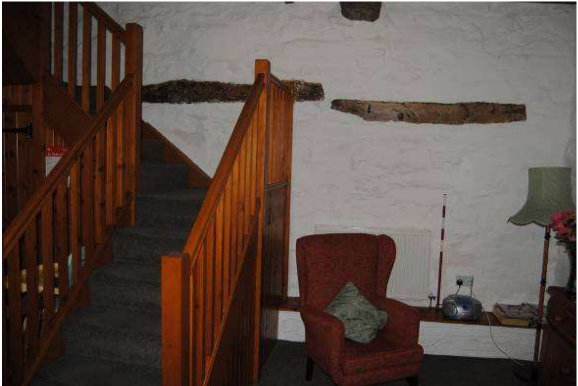
Plate 11: Timber lintels within north wall.
