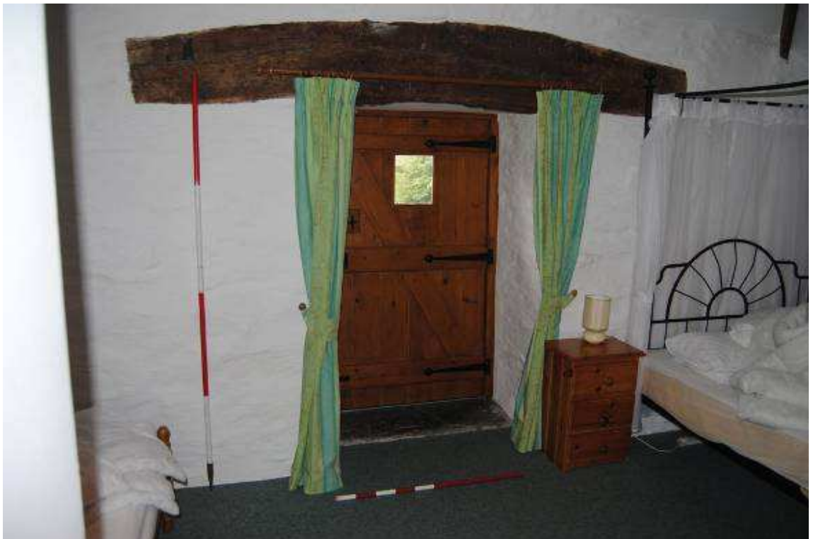
Plate 12: [1F02]; doorway to east gable. NB: oversized lintel (re-used FP bressumer).
