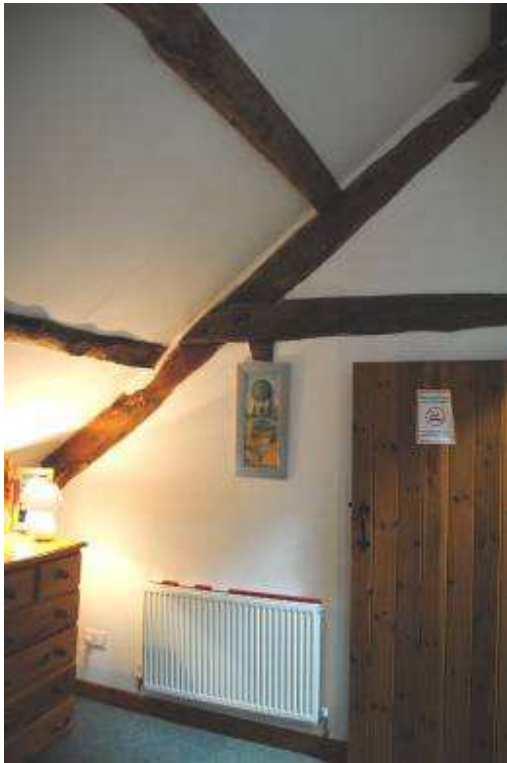
Plate 20: Inserted strut to T2 (south).
