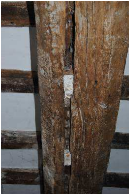
Plate 9: Groove to soffit of beam A.
