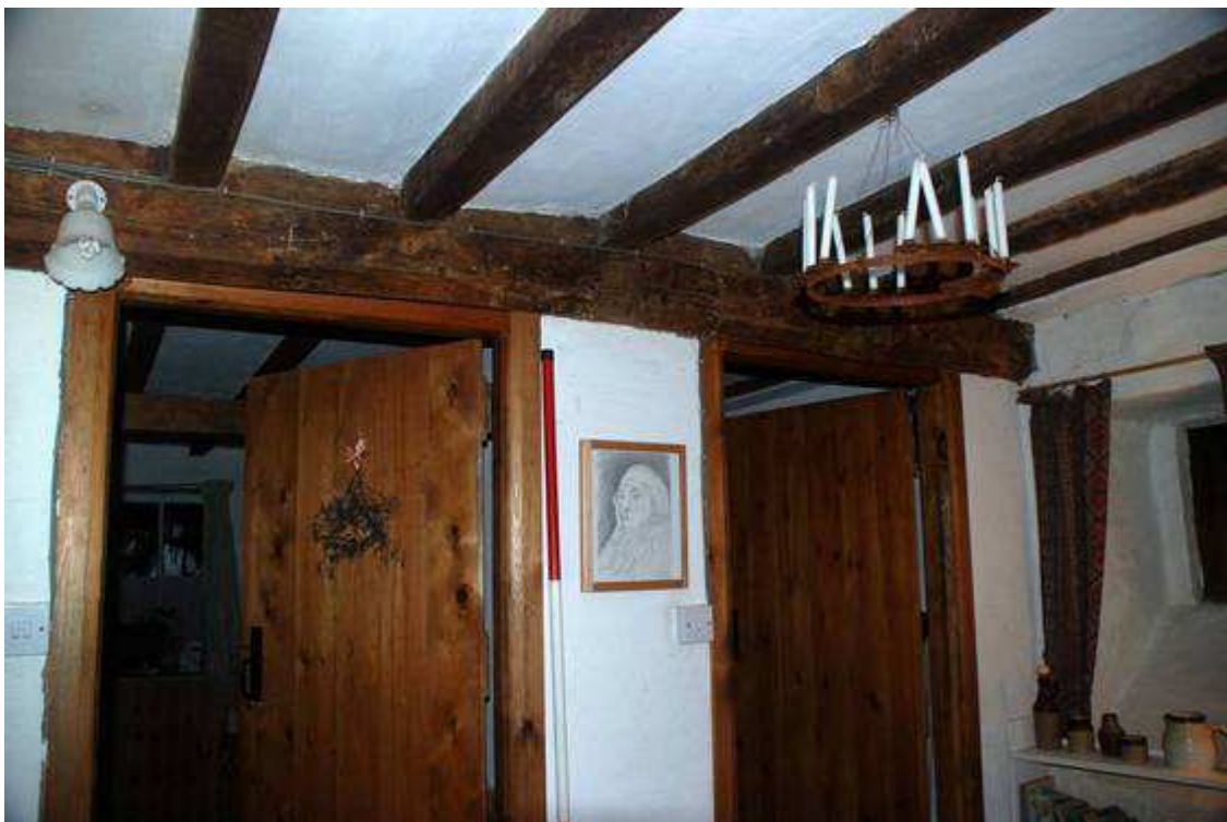
Plate 31: Trenched joists in corridor linking main range to North Wing, looking west
