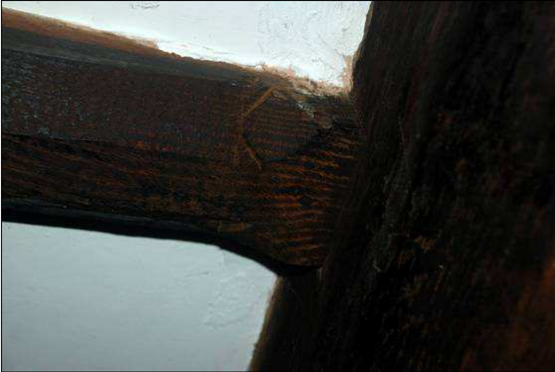
Plate 28: 'Spade' stop on joist in the kitchen
