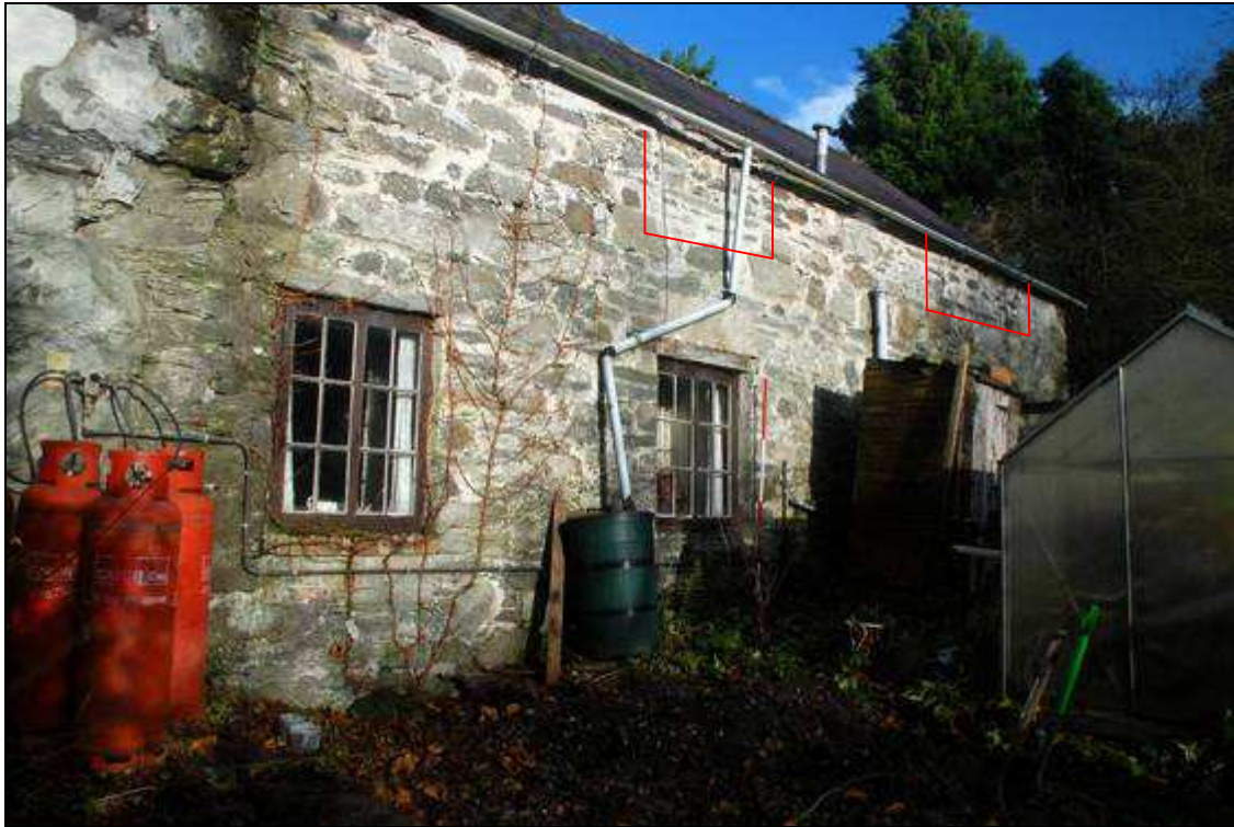
Plate 5: Blocked openings in the southern wing, looking NE
