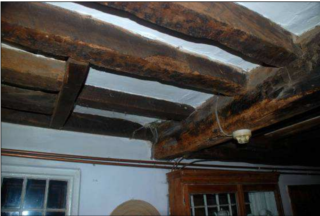
Plate 29: Trimming joist in ceiling of kitchen
