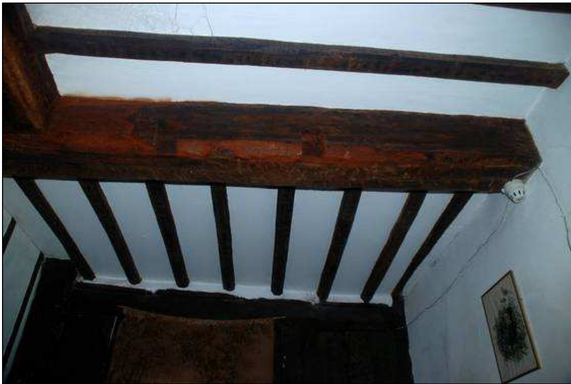
Plate 25: Empty stopped lap joints in longitudinal beam, looking east
