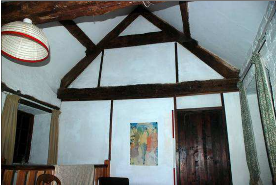
Plate 34: Truss in the North Wing, looking east
