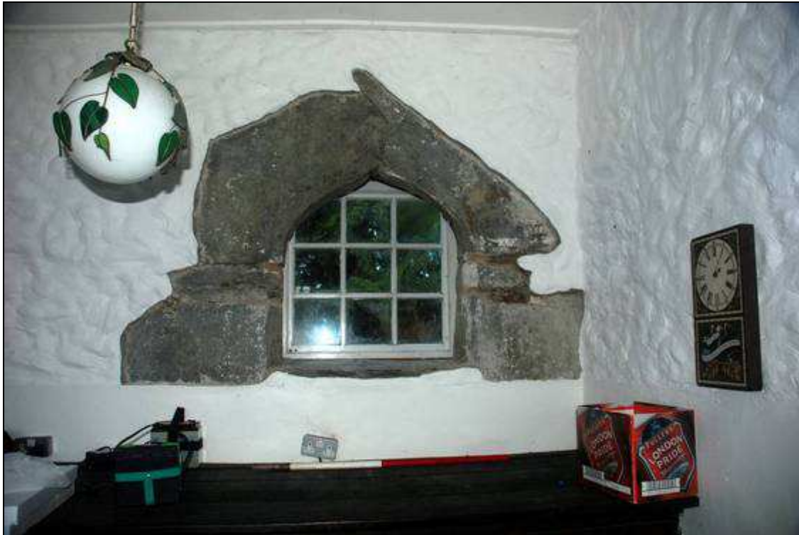
Plate 19: Cyclopean door head in the out building, looking east
