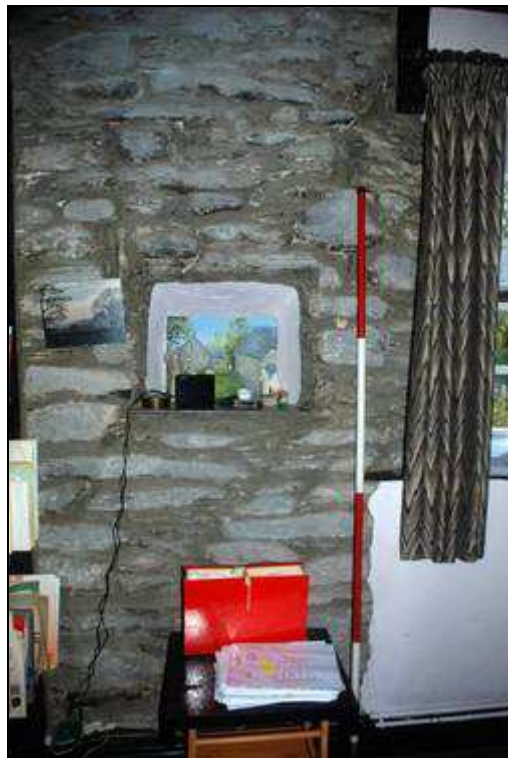
Plate 18: Blocked opening in SW corner of western room, looking west.
