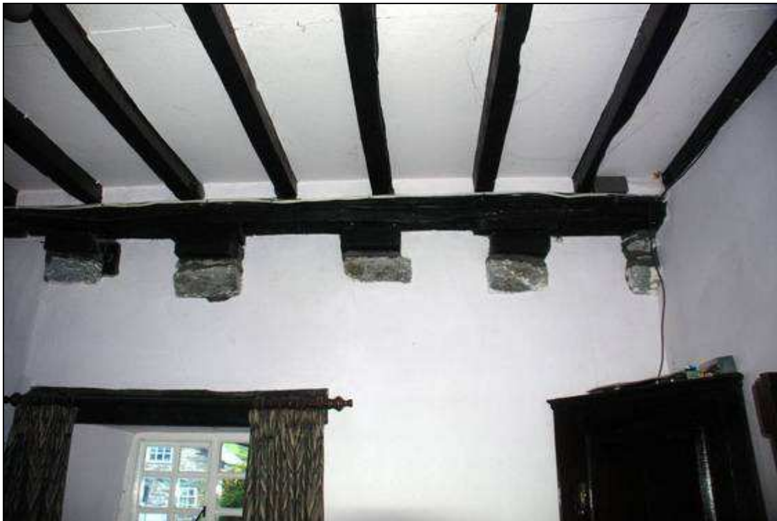
Plate 16: Stone corbels in western wall, looking west
