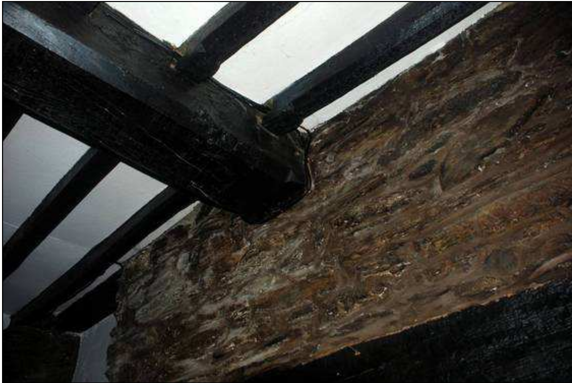
Plate 15: Chamfer and stops on joists and main beam, eastern ground floor room, looking NW
