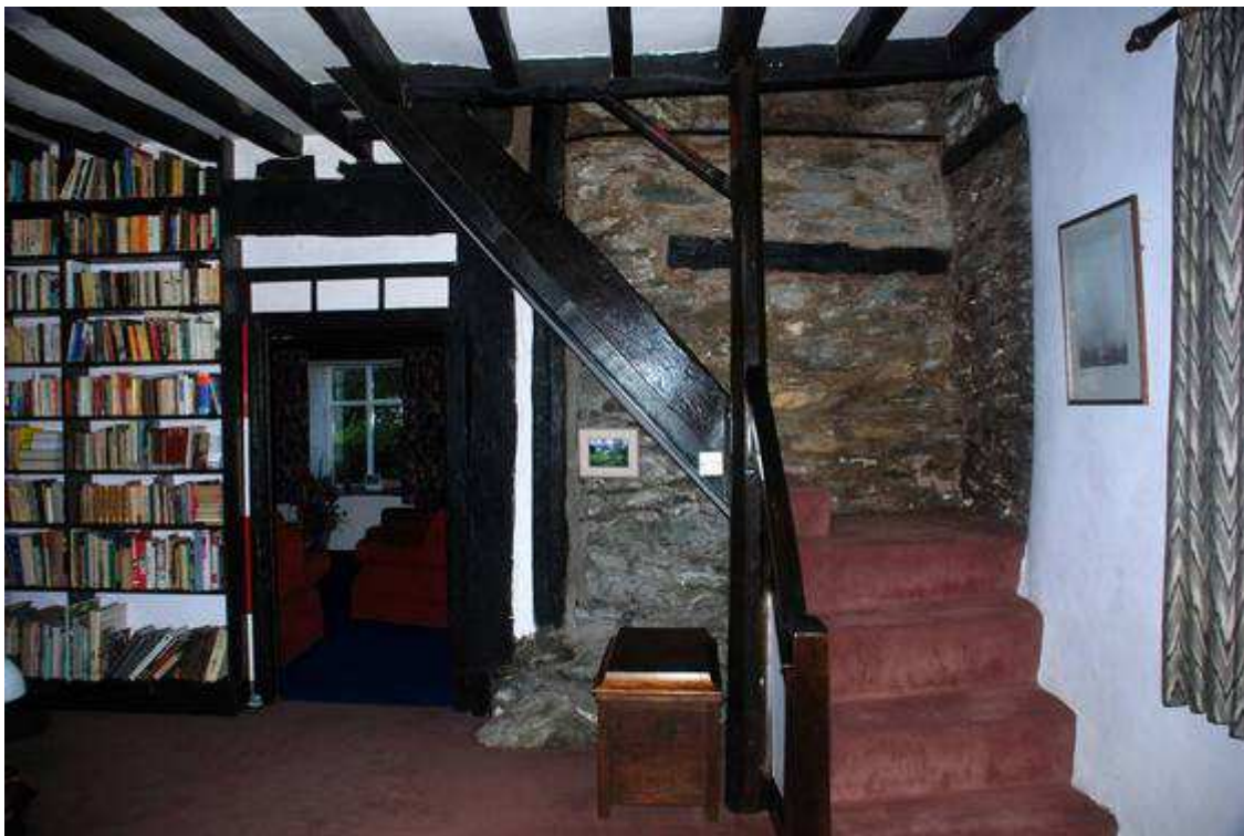
Plate 8: Base of southern post with probable tie-beam, looking east
