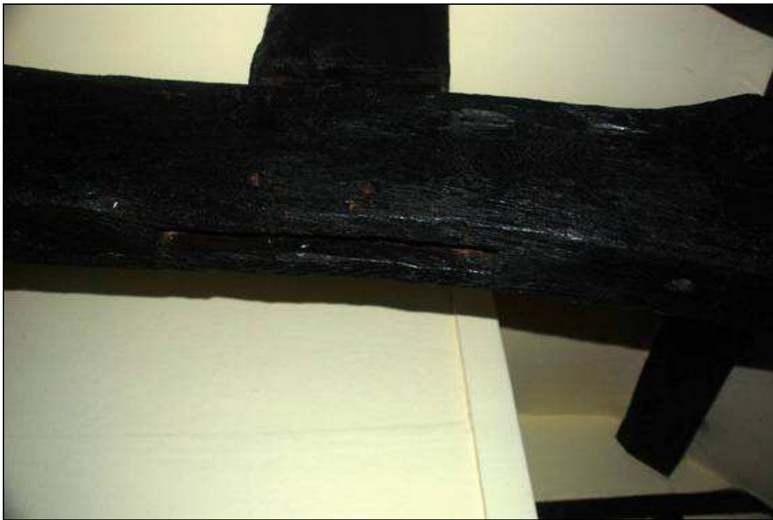
Plate 12: Mortice and dowel holes below Truss 3
