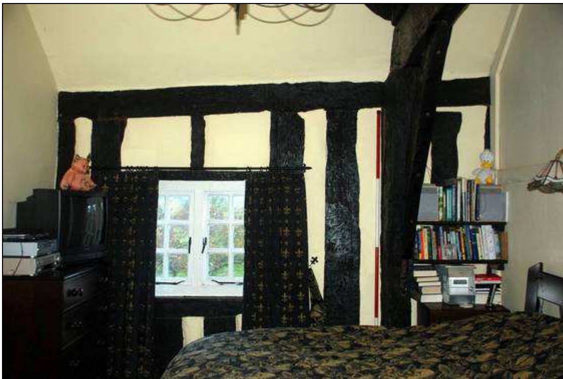
Plate 10: Studwork in the western bedroom, looking north
