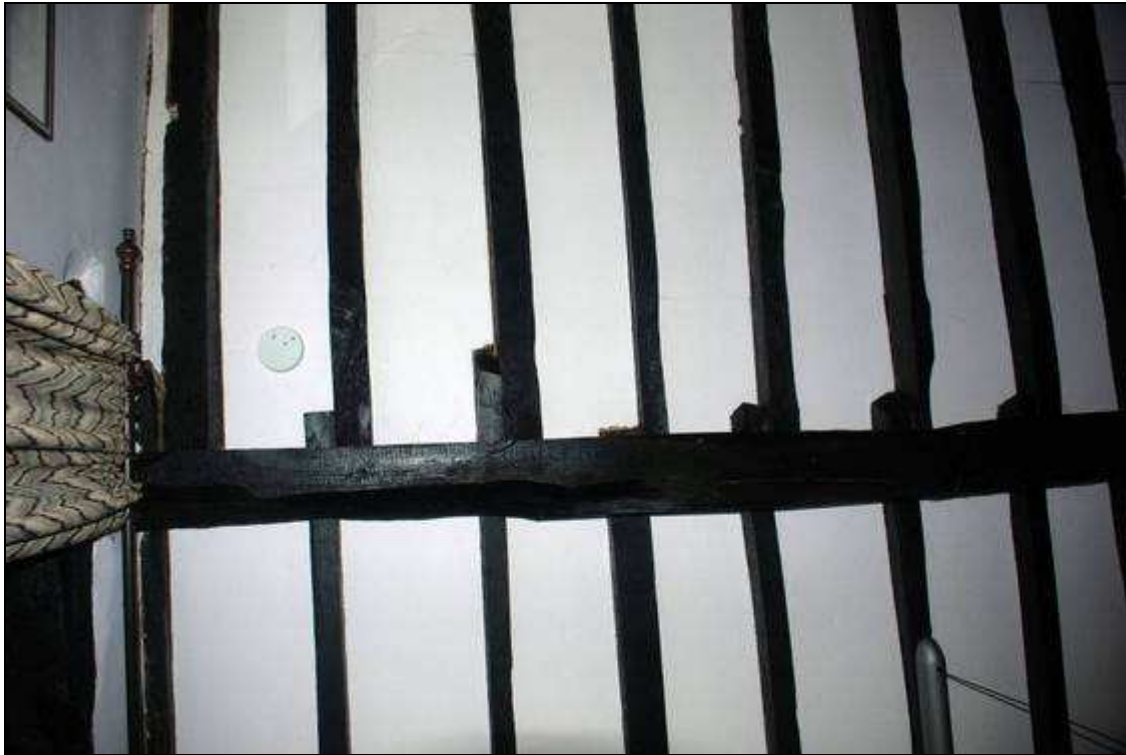
Plate 17: Pattern of main ceiling beam and joists in western room, looking up
