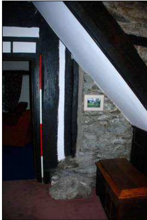
Plate 9: Main southern post and stone projection, looking east
