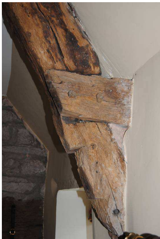
Plate 12: Cruck [T3] (W); truncated tie.
