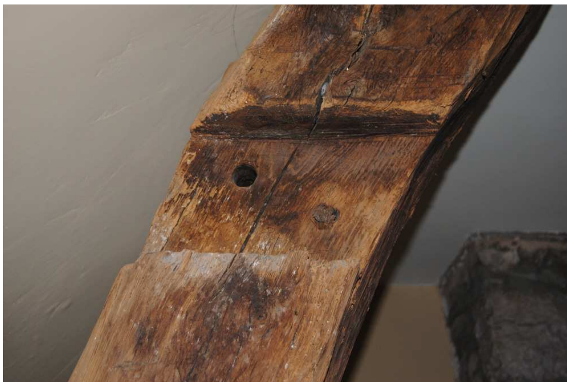
Plate 11: Cruck [T3] (E), redundant lap-joint for tie.
