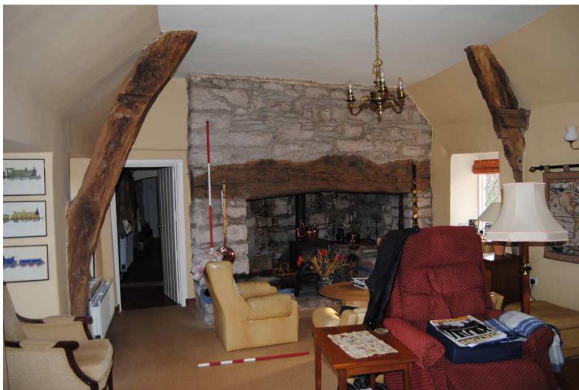
Plate 10: Cruck [T3] looking south towards inserted stack.
