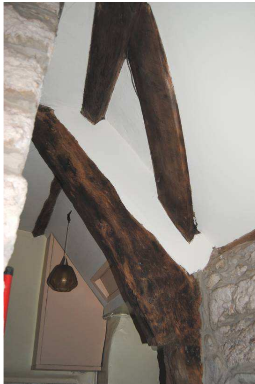
Plate 15: Cruck [T2] (E); wind-bracing to lower purlin.
