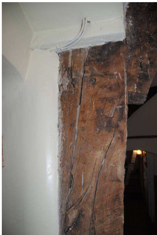
Plate 14: Cruck [T2] (E); detail of post.
