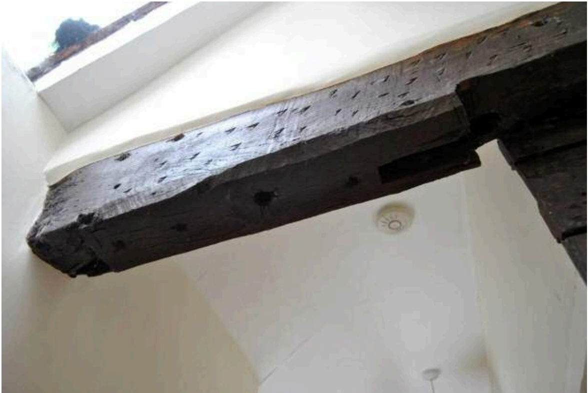
Plate 24: Tie beam of truss TIII at west end of first-floor passage [F2] ; note post-mortice and stave holes to soffit.
