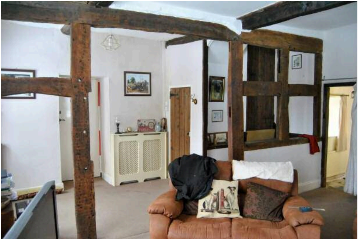
Plate 37: Room [G7] looking north-east with open-framing partition.
