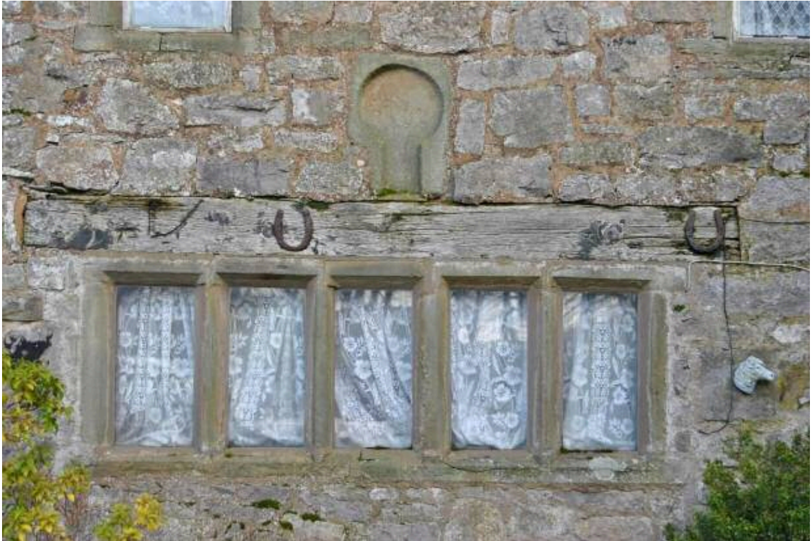
Plate 49: North-eastern extension, east elevation; detail of 5-light window (with lower stone of cheese press over).
