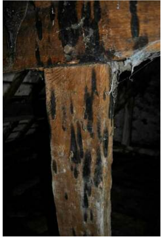
Plate 47: Multiple taper burn marks on QS/collar of truss T1.
