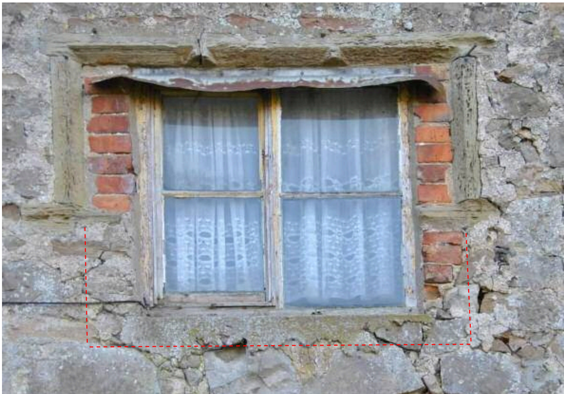
Plate 10: 1F, two-light timber casement inserted into former three-light stone mullioned (and transomed?) opening.
