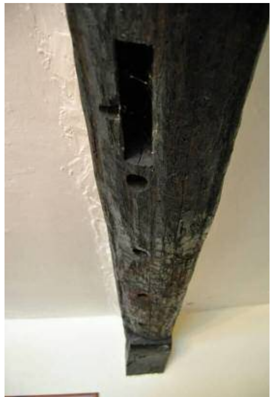
Plate 16: Eastern ceiling beam of [G1] with post-mortice and stave holes for former infill.
