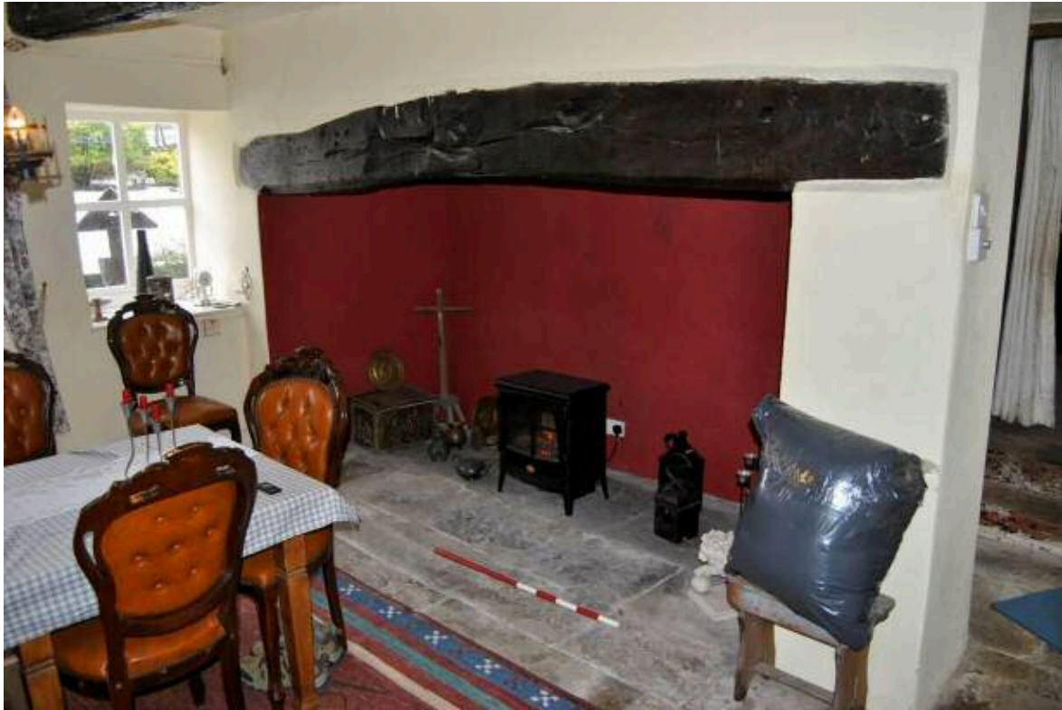
Plate 14: Wide fireplace to west side of [G1] with chamfered, slightly cranked bressumer.
