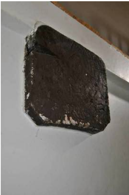
Plate 19: Axial ceiling beam of 'Unit 2', cut through for insertion of Stair B.
