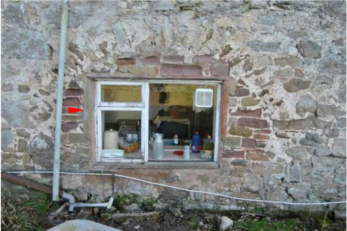
Plate 11: Modern GF window of main range, east gable end, replacing stone mullion window (note jamb to left) and inserted within blocked, arched opening.
