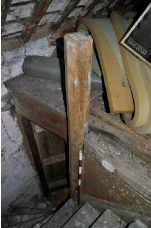
Plate 42: Upper flight of Stair A (1F→attic); detail of octagonal mast-newel.
