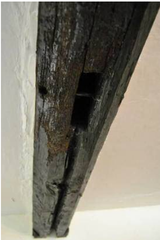
Plate 15: Western ceiling beam of [G1] with post-mortices and groove for infill panel.
