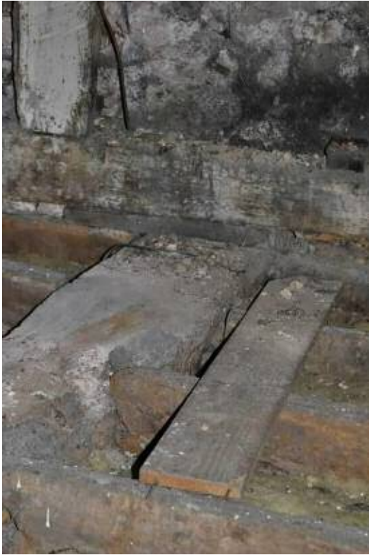
Plate 46: Tie beam of T11 sits atop axial ceiling beam.
