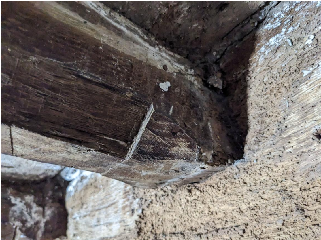
Fig. 9 – Chamfer and stop detail in outer room.
