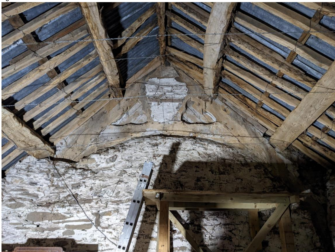
Fig. 6 – Central cruck to hall; cusped trefoils survive, but note the lefthand missing cusp, which was never formed.
