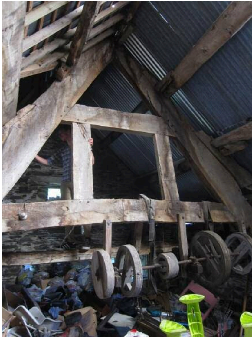
Fig. 1 - Cruck truss T1 with equipment associated with the Pelton water wheel.
