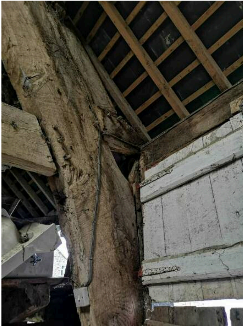
Fig. 3 - Detail of horn and packing piece.
