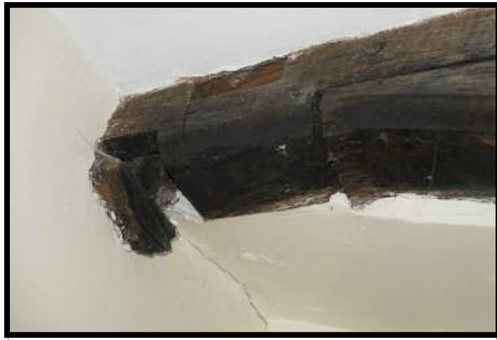
Figure 18: Bottom of principal with stud and mortise.
