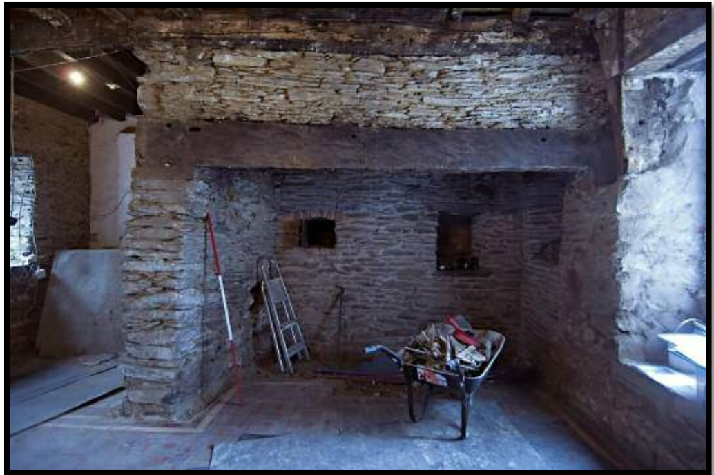
Figure 11: Inserted fireplace in hall.
