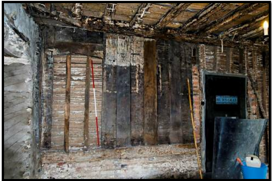
Figure 9: Remnant of plank & muntin screen.
