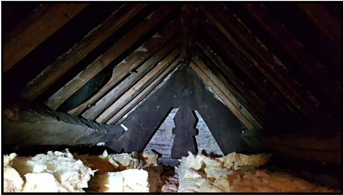
Figure 20: Unusual decorated king strut on Truss 1
