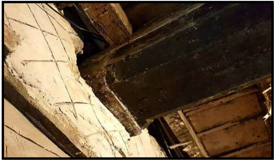
Figure 15: Main transverse beam with chamfers and stops.
