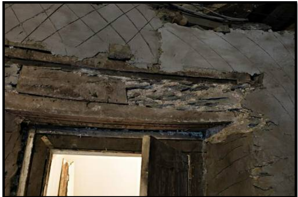
Figure 14: Re-used timber - rebated rails, holes and oddments.
