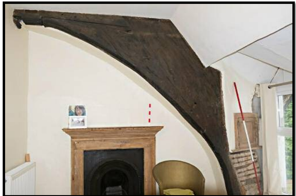
Figure 16: Right blade of Truss 1. Arch-braced.
