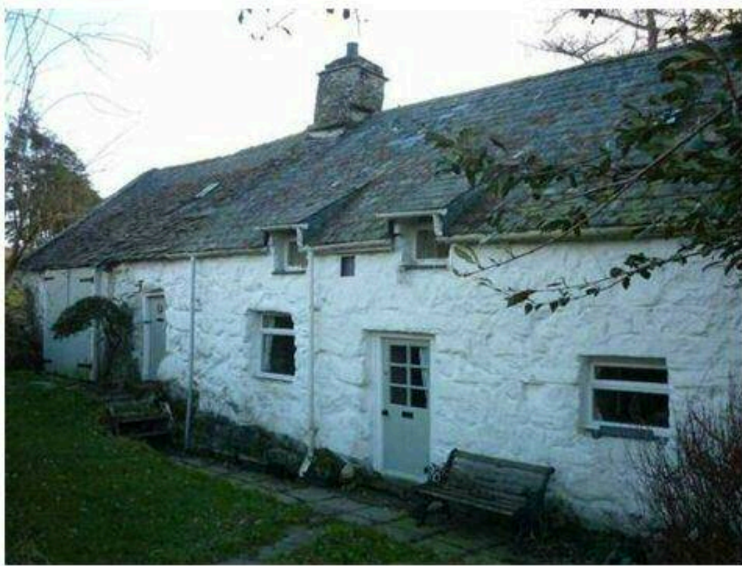
3. East elevation, south end.
