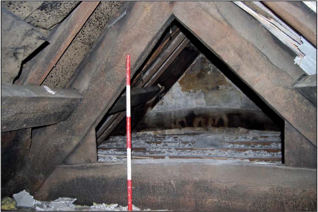
Plate 3: South facing image of truss 4.
