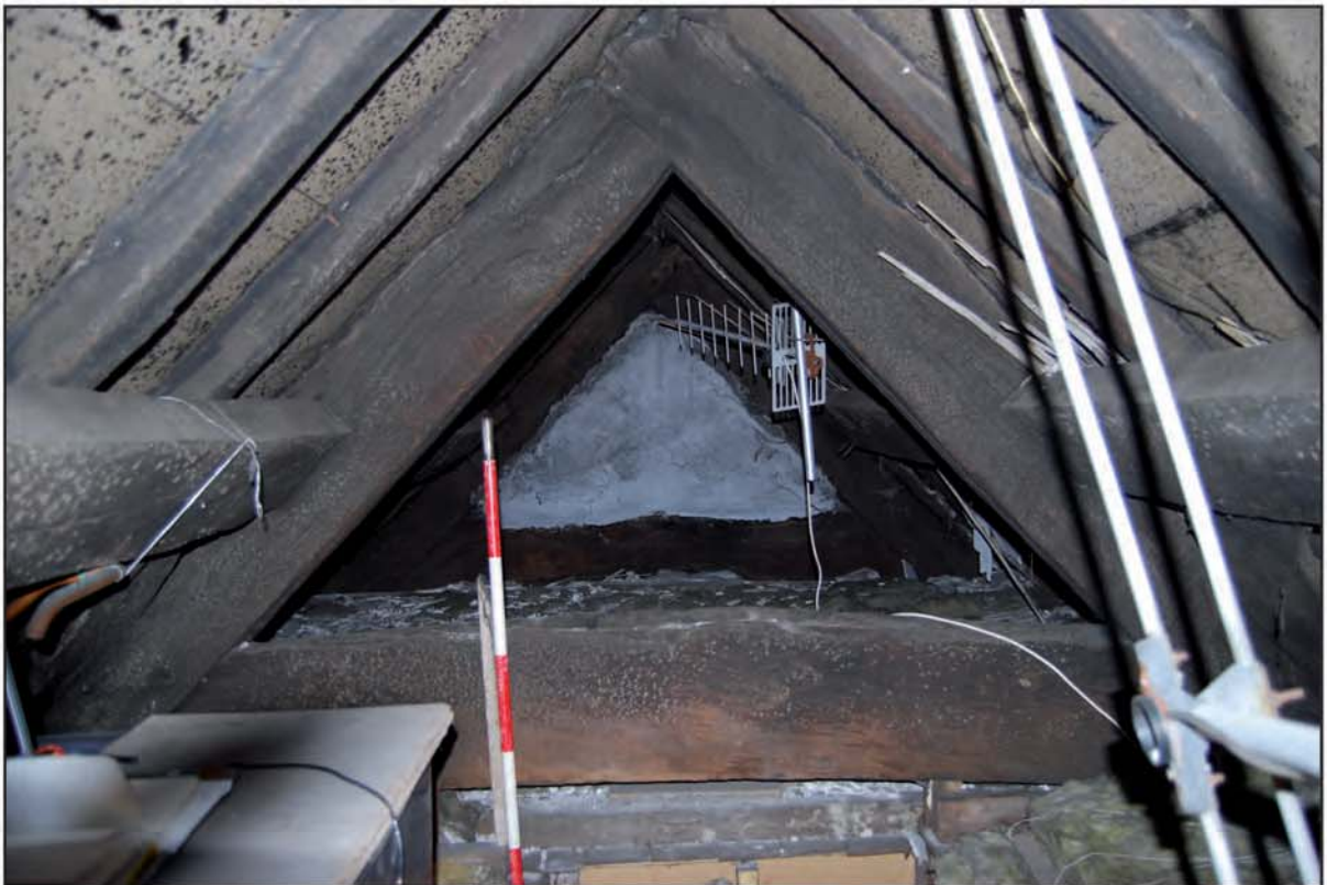
Plate 4: North facing image of truss 2 & 3.
