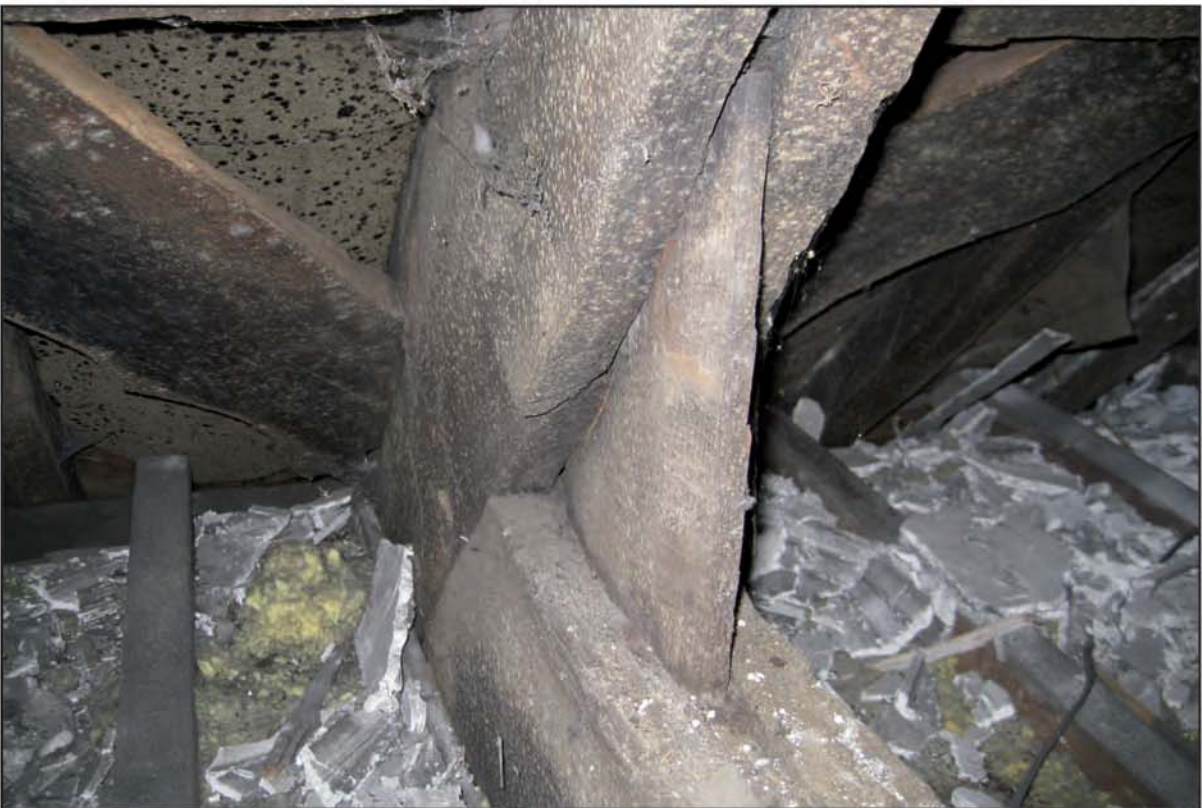
Plate 6: South-west facing image of section of oak planking in truss 4 showing chamfer on the outer edge.
