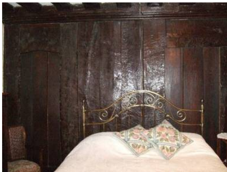
Post and panel partition in the solar
