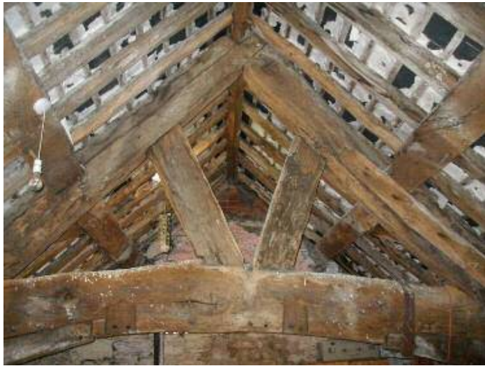
Arch braced collar with raking struts
