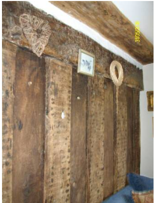
Plank and Muntin wall panelling also known as a post and panel partition
