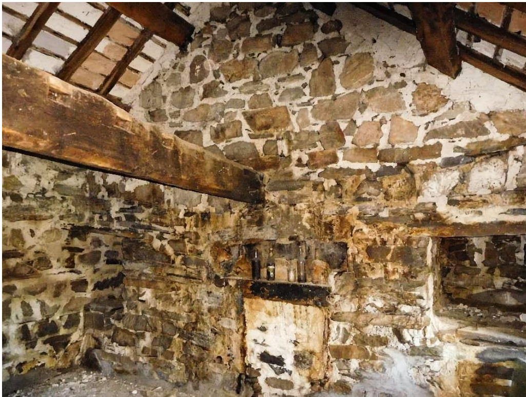
Above : Inside gable wall of rear part of Llenyrch (Jenny Lees 2023)
