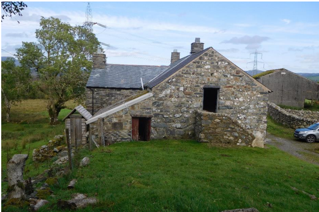
Above: Llennyrch - gable end of attached barn and granary (Jenny Lees 2023)
