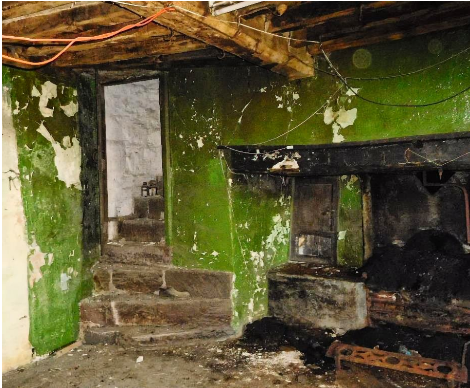
Fireplace stair and left part of huge bressumer at Llennyrch (Jenny Lees 2023)
