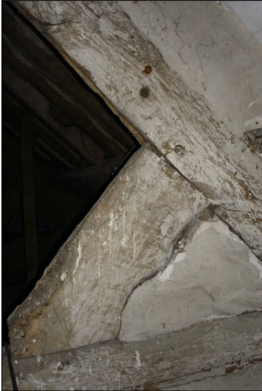
Figure 3: Detail of western side of reused cusped truss T2 showing ill-fitting joint to principal rafter
