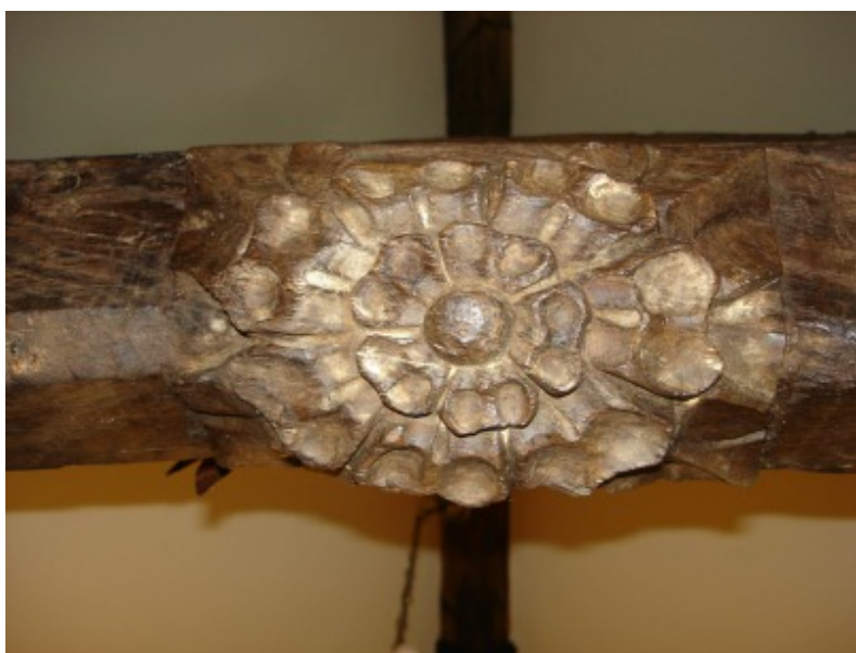
Figure 2: Photograph of carved boss to open truss
