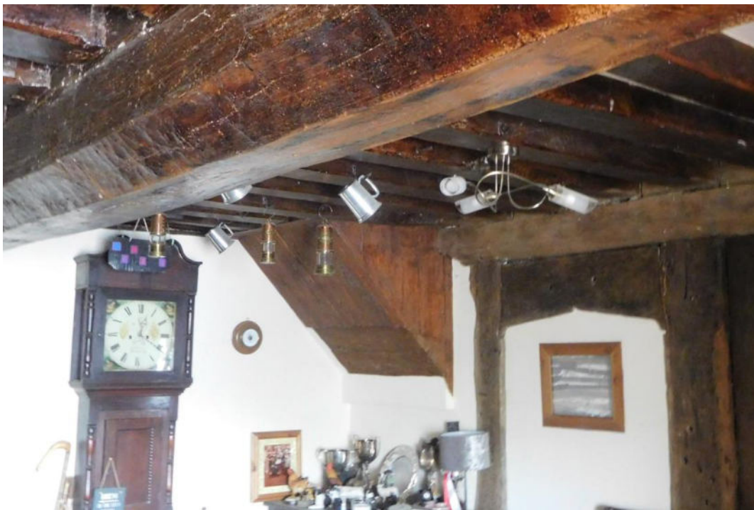
Northeast corner of ground floor room at Caenog, with north end of ‘post and panel’ screen
