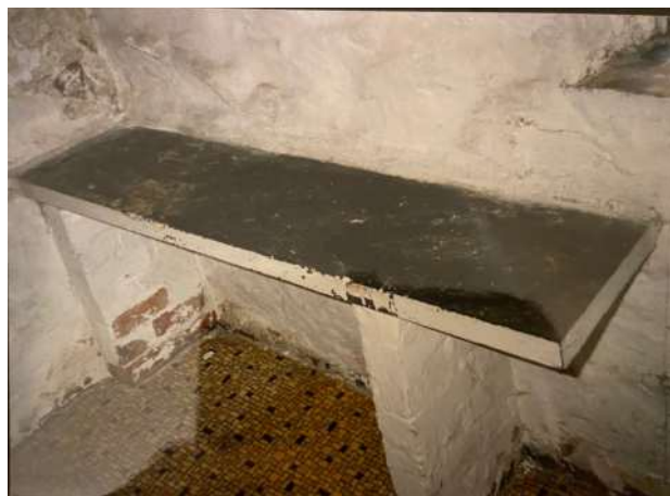
The slate slab in the scullery.
