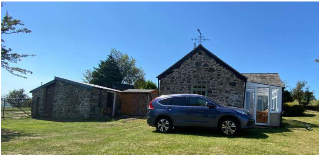
The bakehouse was the building on the left of the picture.
