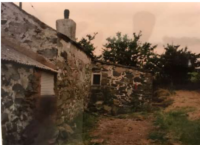
The small section which is jutting out from the back was a scullery which would have been a later addition.
