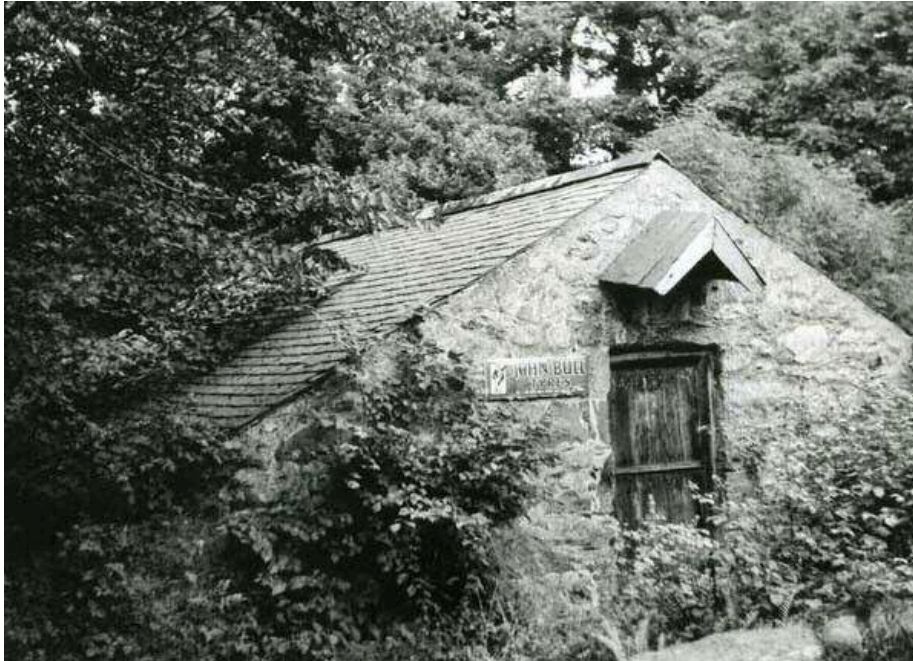
The top storey of the mill at ground level 57
