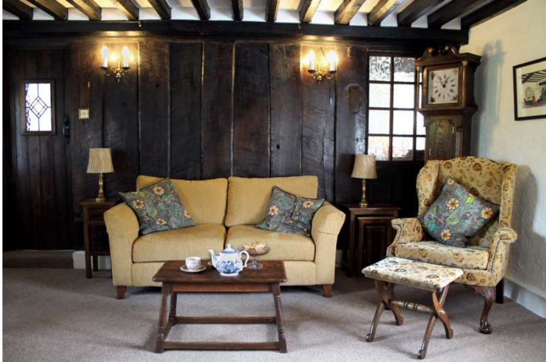
Oak post-and-panel dais partition at Henfaes isaf (Image courtesy of Moyra James)
