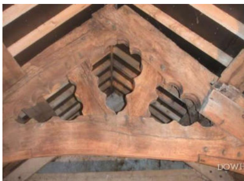
Trefoil Roof Truss
