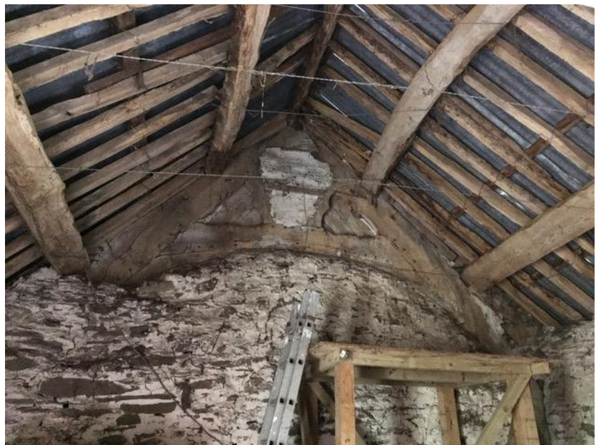
Hafod yr Afr, Cynwyd, Denbighshire The principal hall truss tree-ring dated to c.1533-63
