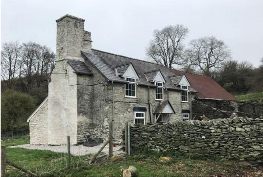
Hafod yr Afr, Cynwyd The open hall survives under the corrugated iron roof
