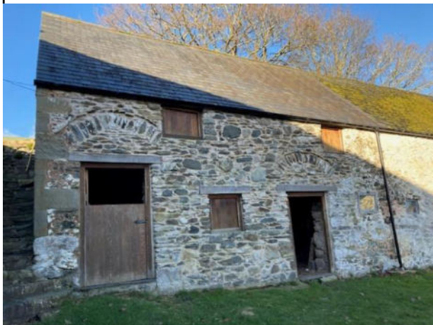
The Dovecote (the external staircase is to the left)
