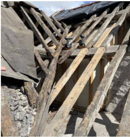
Repairs in reclaimed oak to the roof valley timbers
