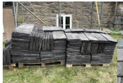
Thick Welsh reclaimed slates arrive from South Wales complete with lichen
