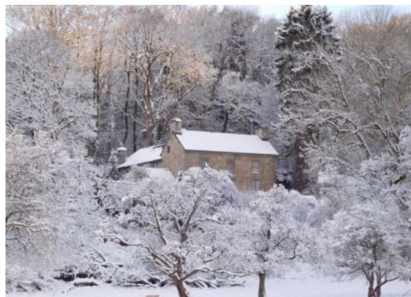
Hafod y calch Georgian east wing with pre C17th parts behind to the left
