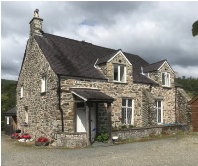
Y Faner from the SW, close to the perimeter wall of Cymer Abbey. The door leads into the end cross passage - the house appears never to have extended to the left. The open hall (the floor was inserted in c. 1900) is to the right.
