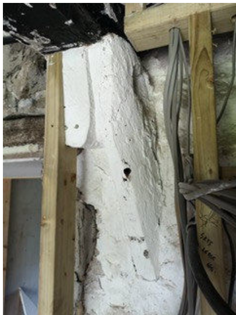
Fig 2 Cwm Mynach Canol - the in-situ stub of a cruck blade (now concealed) that was felled in the spring of 1573 @ Ross Cook, ArchaeoDomus
