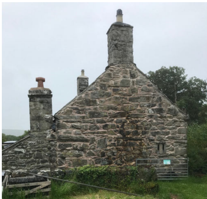
Llwyn Hwlcynd end elevation with the small window that lights the stone spiral mural stair which survives intact.
