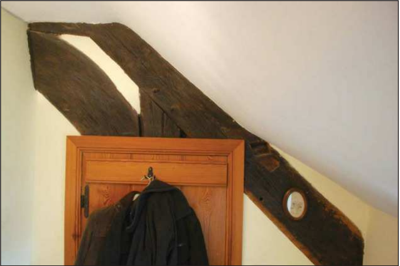
Plate 7: The eastern side of the southern face of the central cruck which forms the south side of the screens passage; view from the south.
