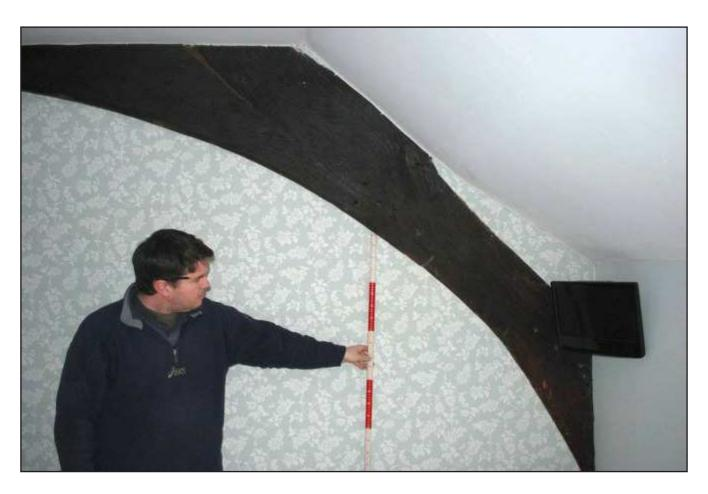
Plate 3: The eastern side of the southern face of the southern cruck which divides the hall; view from the south.
