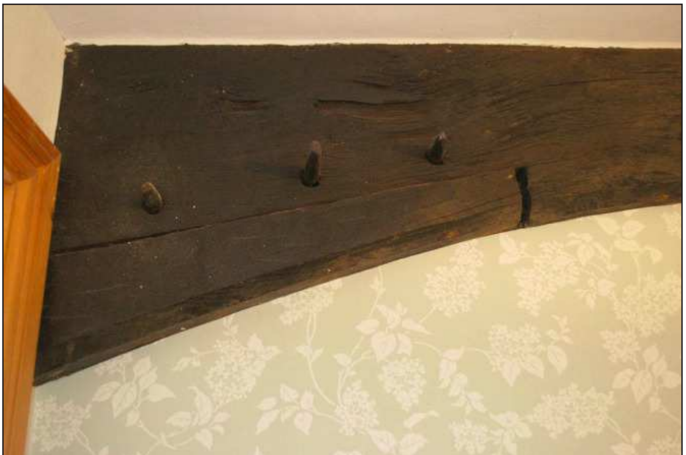
Plate 4: Close up of the pegs which join the jointed vertical post with the principal to form the bend of the southern cruck. This is the western side of the southern face; view from the south.
