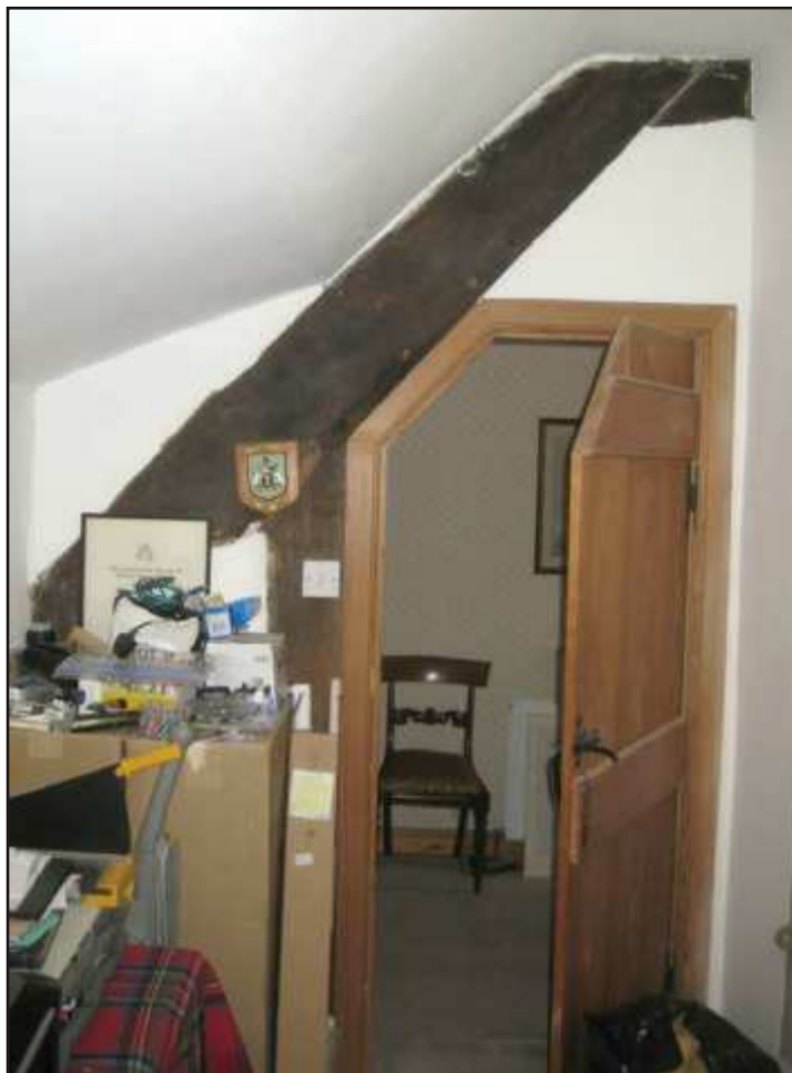
Plate 08: The western side of the southern face of the central cruck which forms the south side of the screens passage
