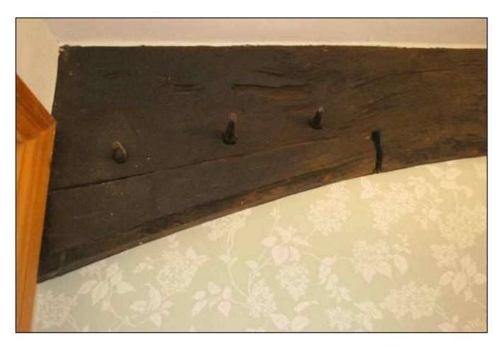
**Plate 4:** Close up of the pegs which join the jointed vertical post with the principal to form the bend of the southern cruck. This is the western side of the southern face; view from the south.
