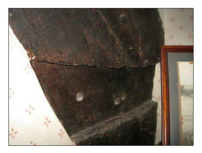
Plate 12: Close up of the housing for a tie beam on the eastern side of the southern face of the northern cruck, which forms the southside of the screens passage; view from the south.
