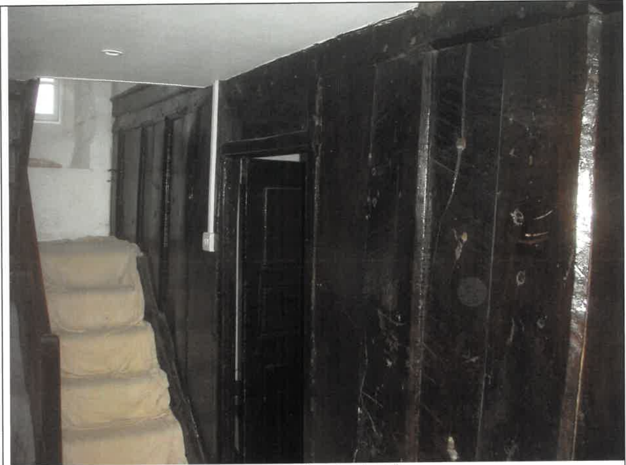
Plate 4 Partition (north end)
