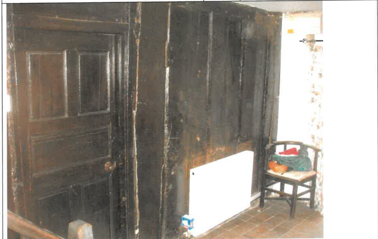
Plate 5 Partition (S end)
