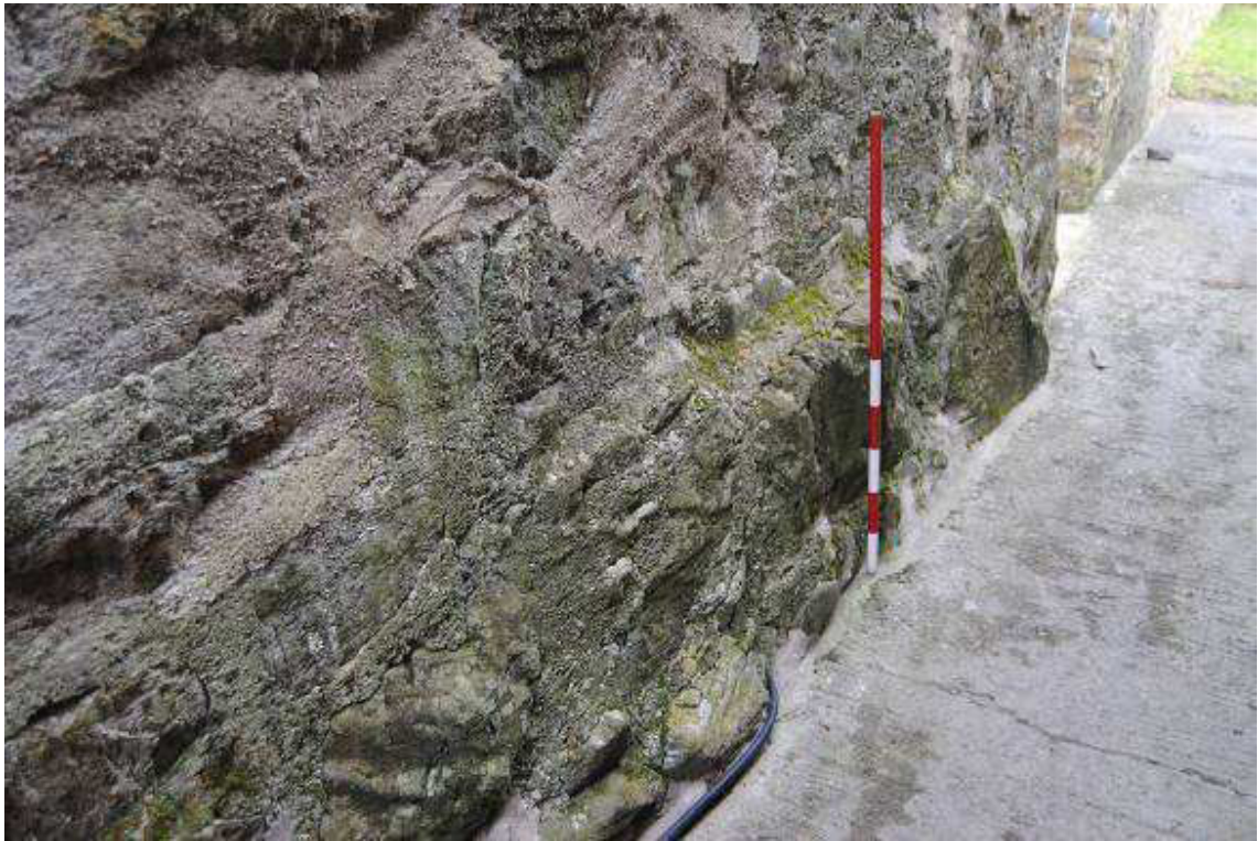
Plate 7: Offset boulder footings to south elevation (also present to east and north elevations and evidenced to west).
