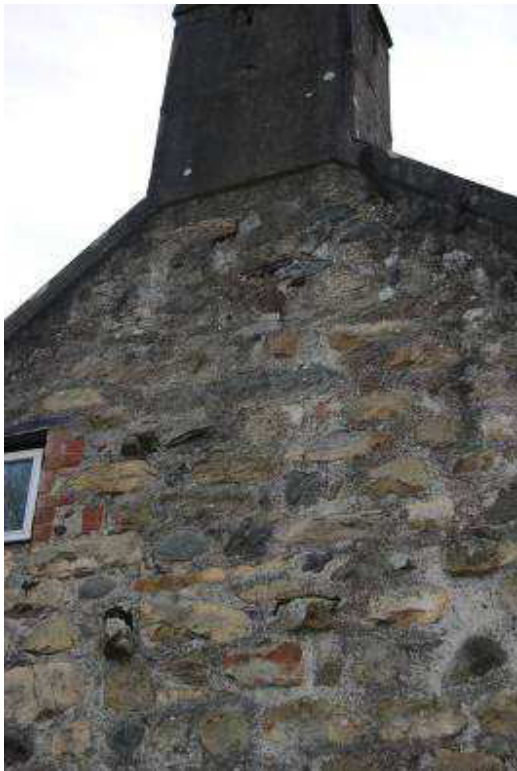
Plate 5: Evidence for possible former corbelled stack to north gable.
