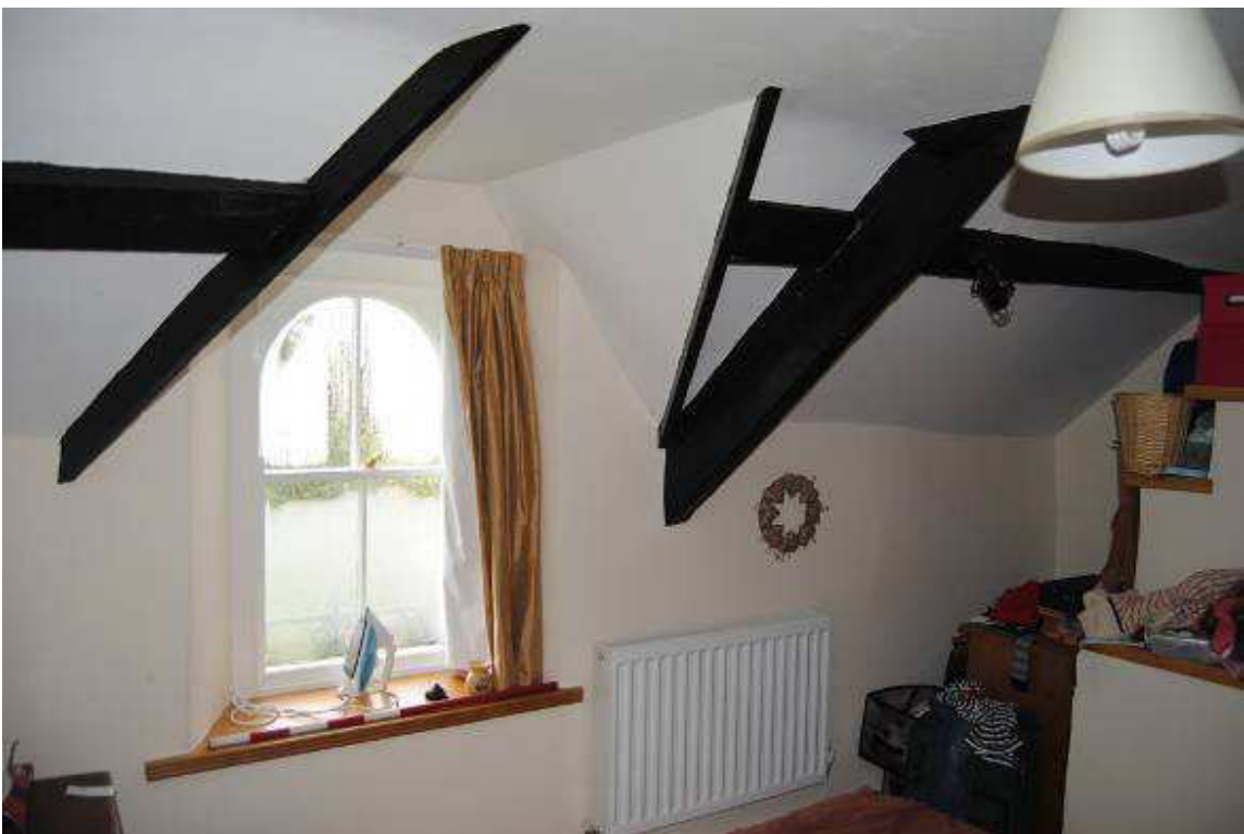
Plate 23: Principal rafter of Truss T1 within Room [1F02] with C19th dormer to left.
