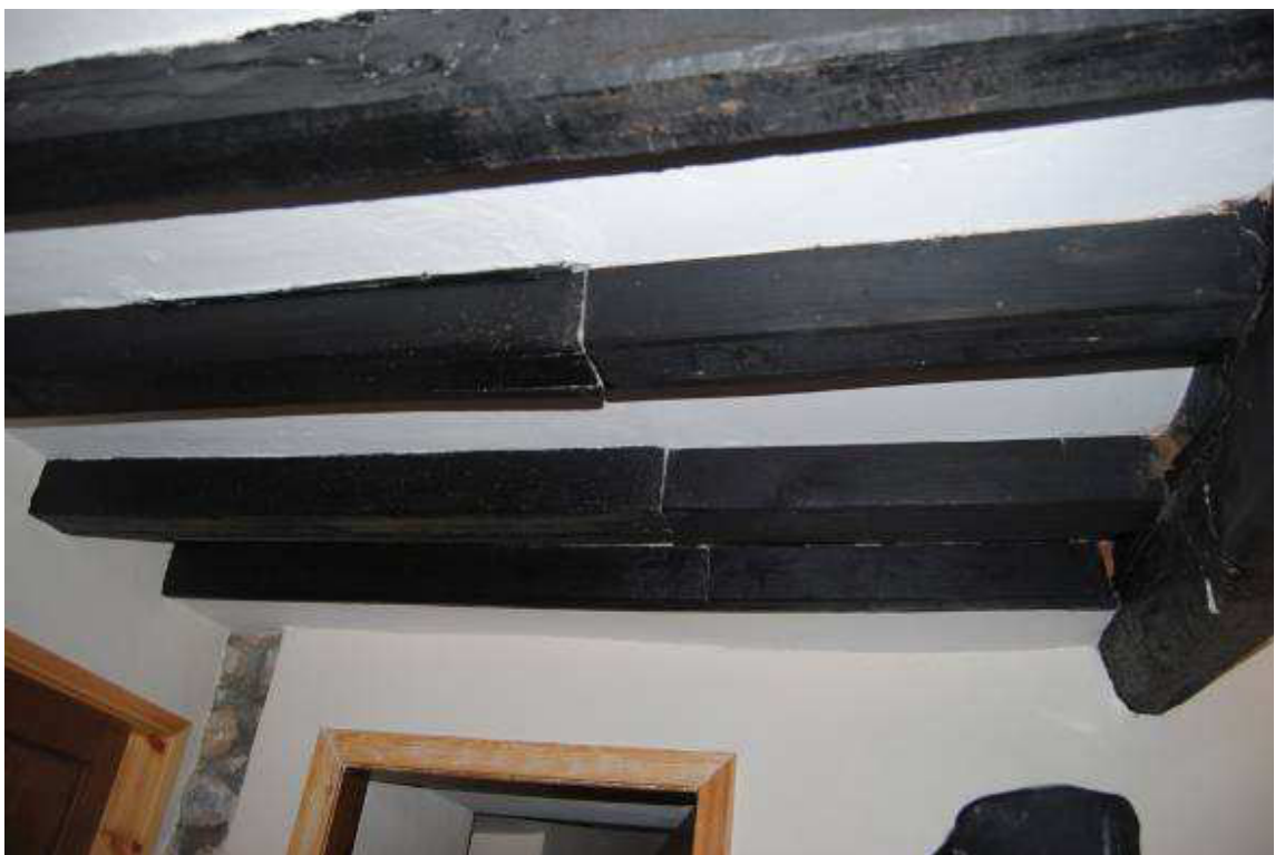
Plate 17: Room [GF02]; renewed ceiling joists to west.
