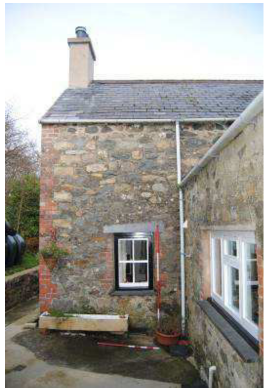
Plate 28: NW extension, south elevation.
