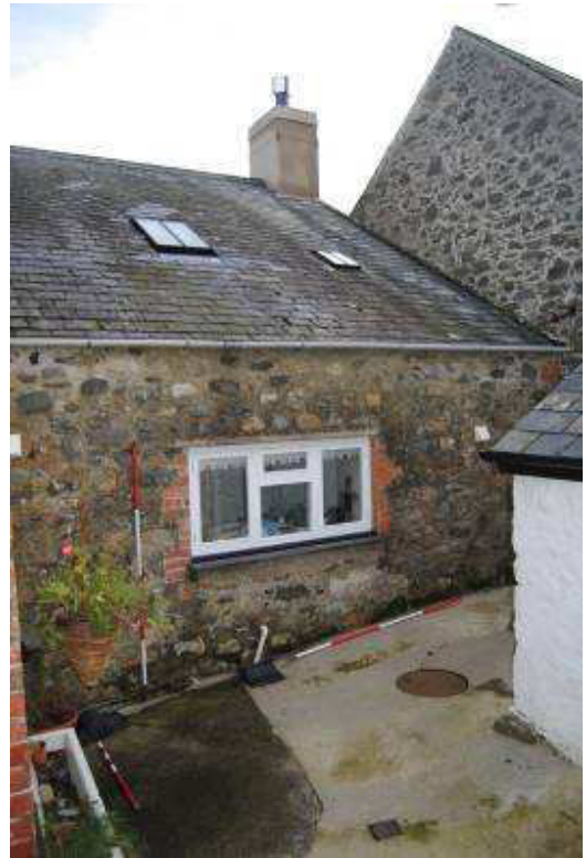
Plate 33: Phase II extension with cat-slide roof.
