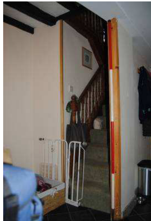
Plate 14: Inserted stair at SW angle of principal range.
