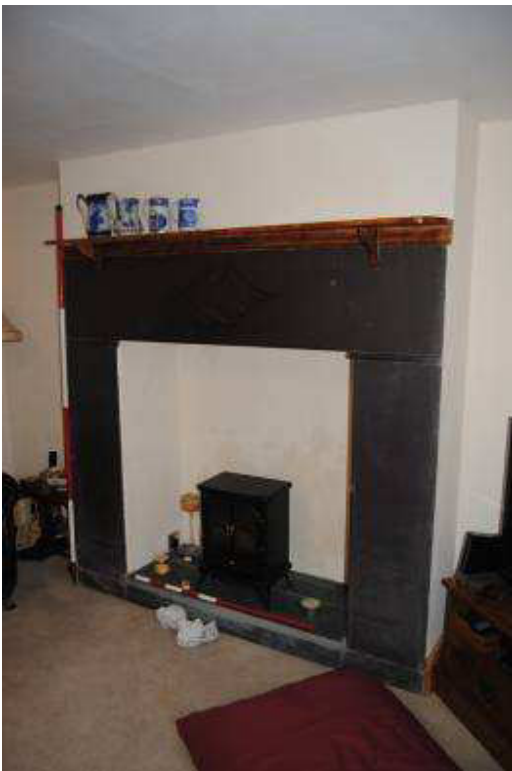
Plate 30: [GF03]; detail of slate FP surround.
