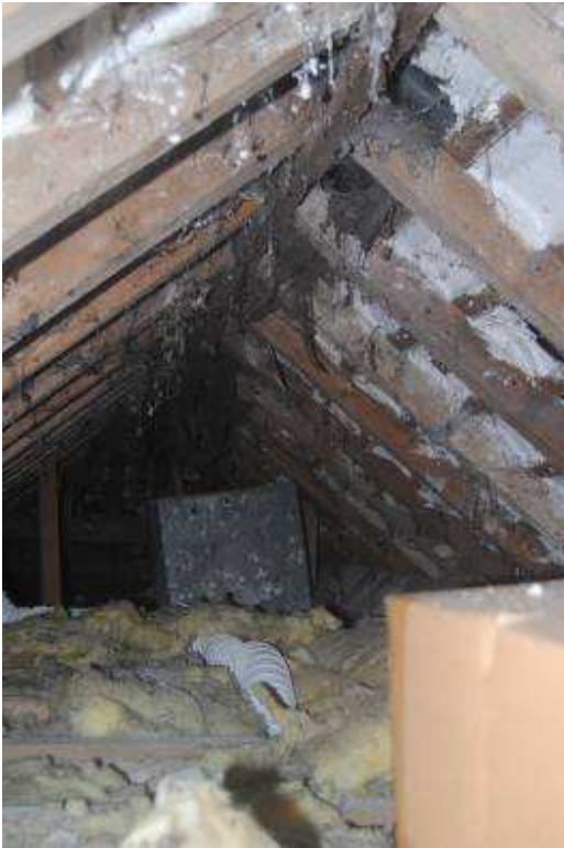
Plate 32: Common rafter roof over NW extension.
