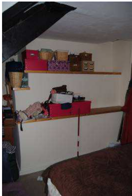
Plate 22: Principal stack within Room [1F02].
