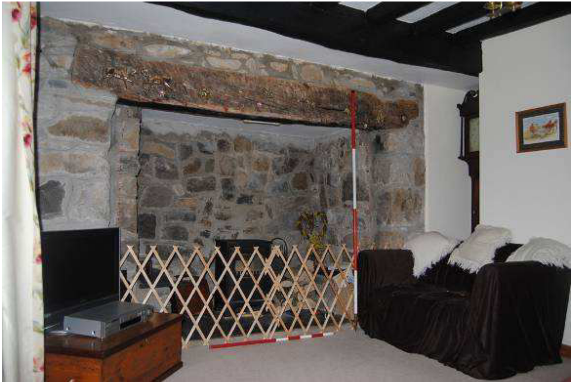
Plate 9: Room [GF01]; principal FP to south wall.
