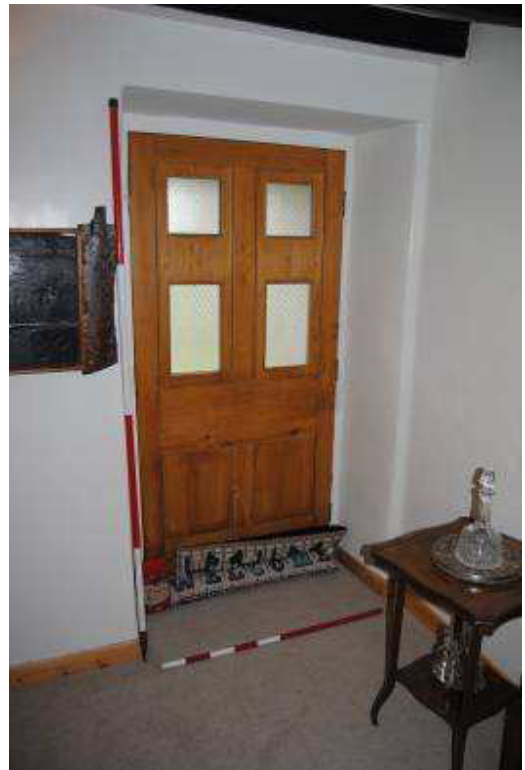
Plate 16: Room [GF02]; door in east wall.
