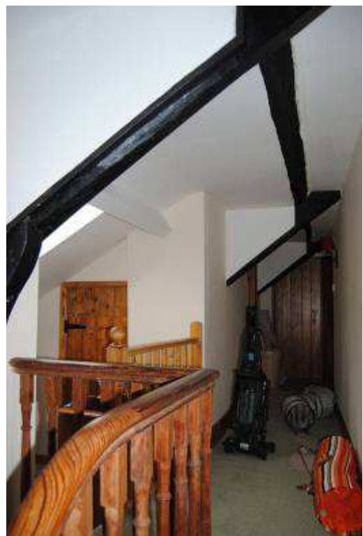
Plate 20: Lateral corridor [1F01] to west side of principal block, note principal rafters.
