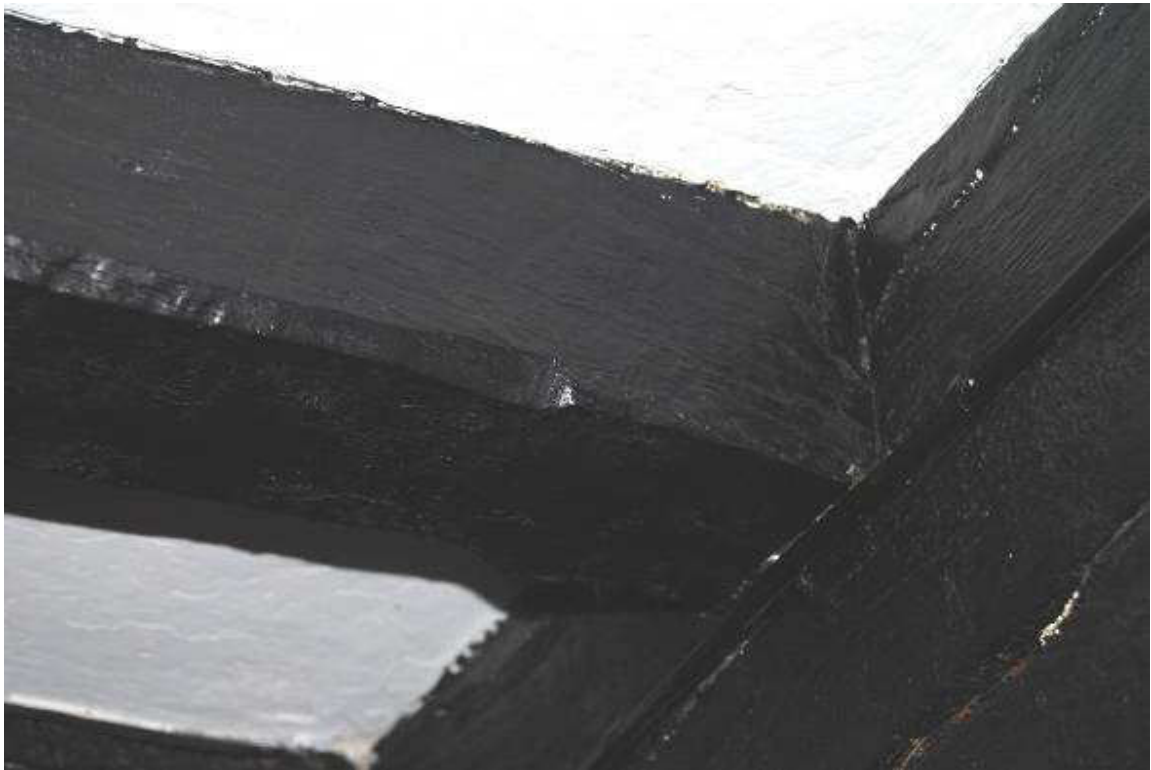
Plate 12: [GF01]; detail of main beam / common joist. NB; fine chamfer, stop and bare-faced soffit tenon joint.
