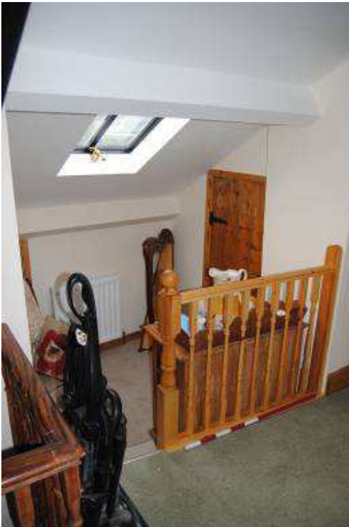
Plate 21: [1F08] within roofspace of SW block
