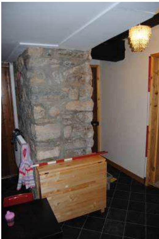
Plate 13: [GF04] truncated west wall.
