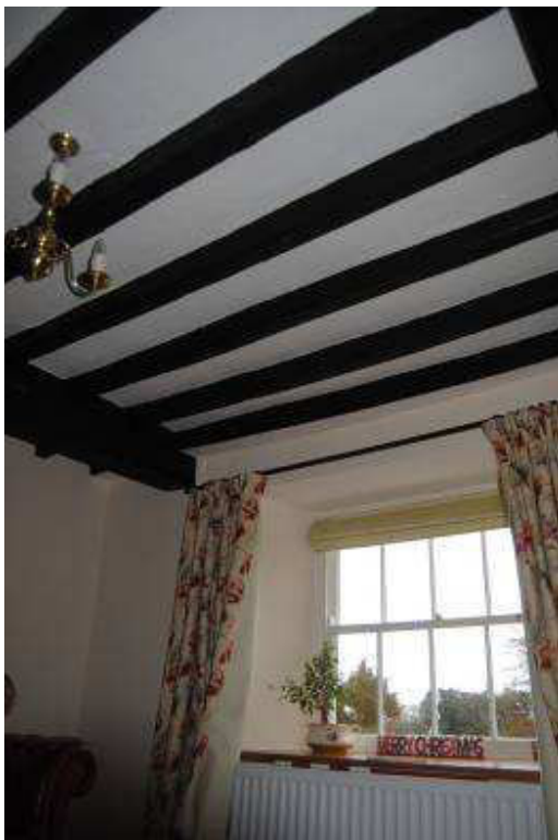
Plate 10: [GF01] ceiling structure, looking east.
