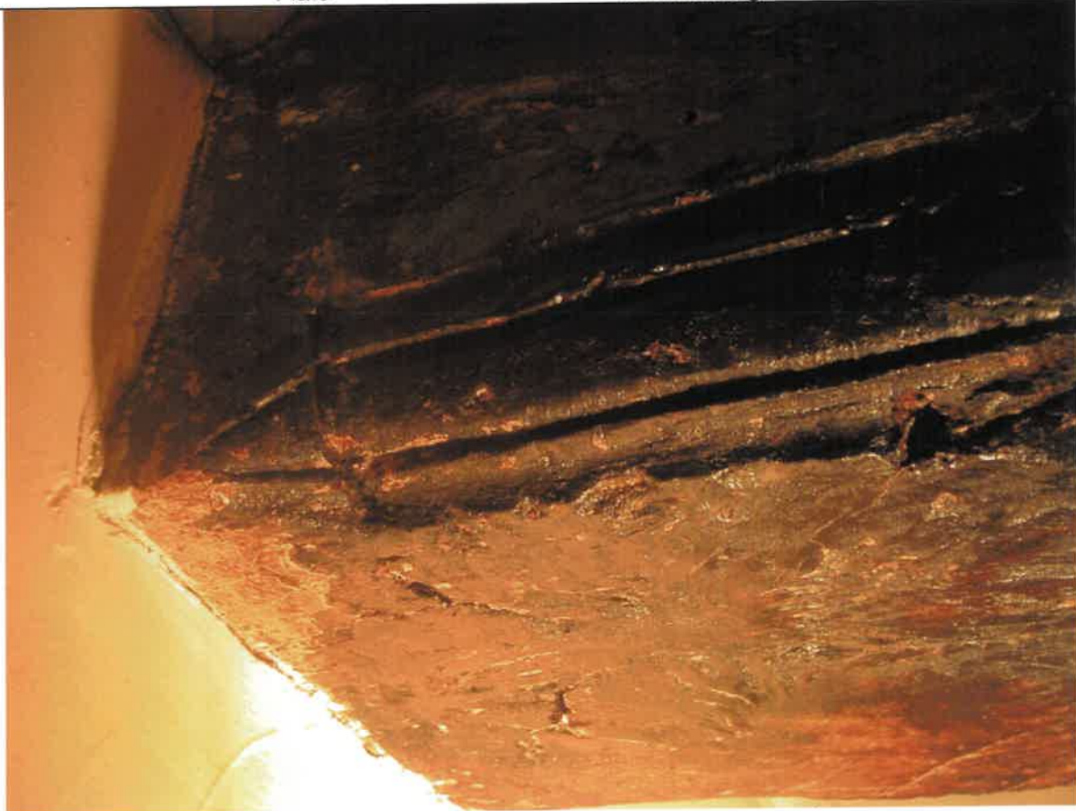
Plate 13 Stop to main beam (west end, south side)
