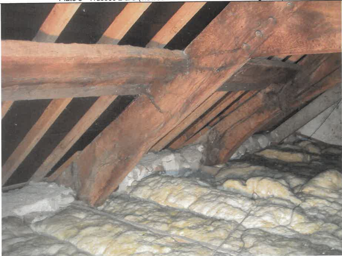
Plate 6 Trusses 2 & 3 (viewed from north - Truss 2 in foreground)
