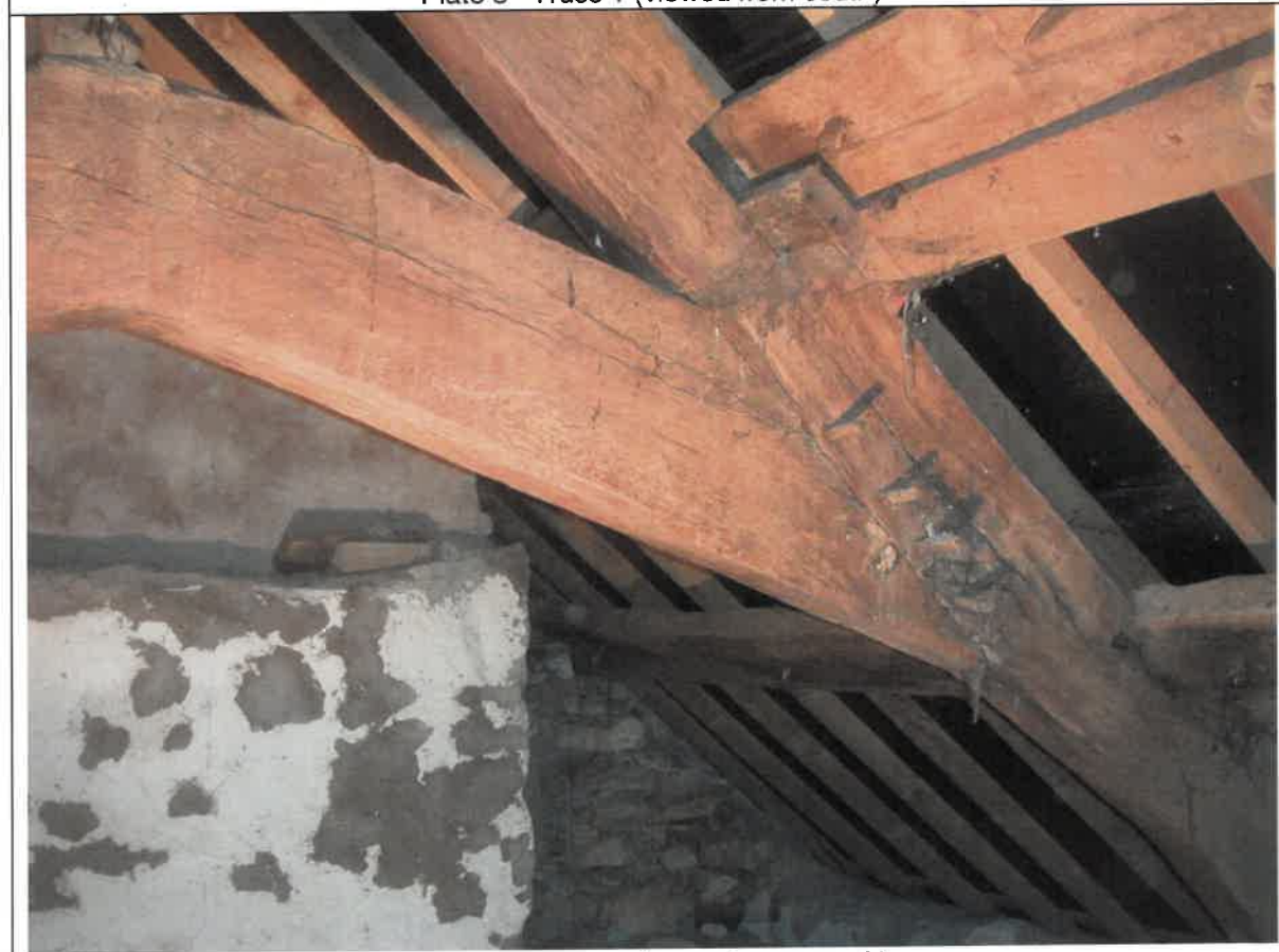
Plate 4 Truss 1 (viewed from south)
