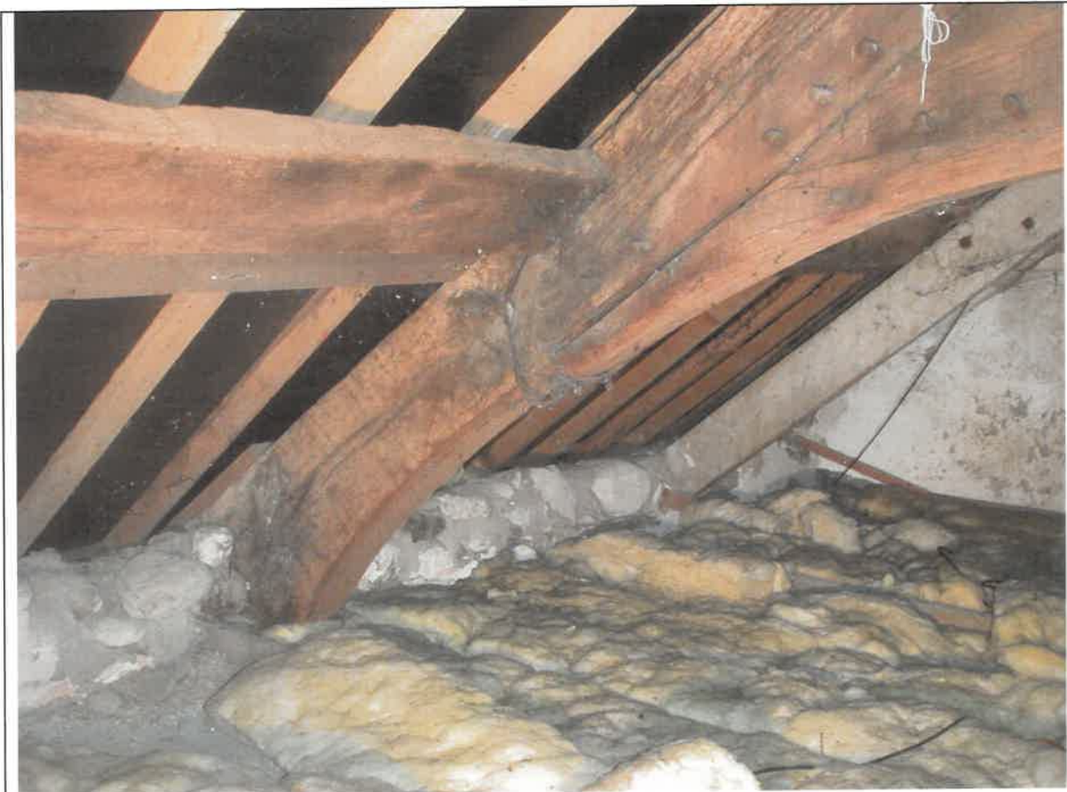
Plate 7 Truss 3 (viewed from north)
