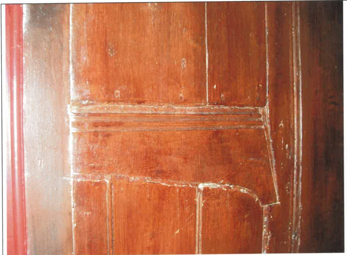
Plate 10 Partition (part of blocked doorhead)
