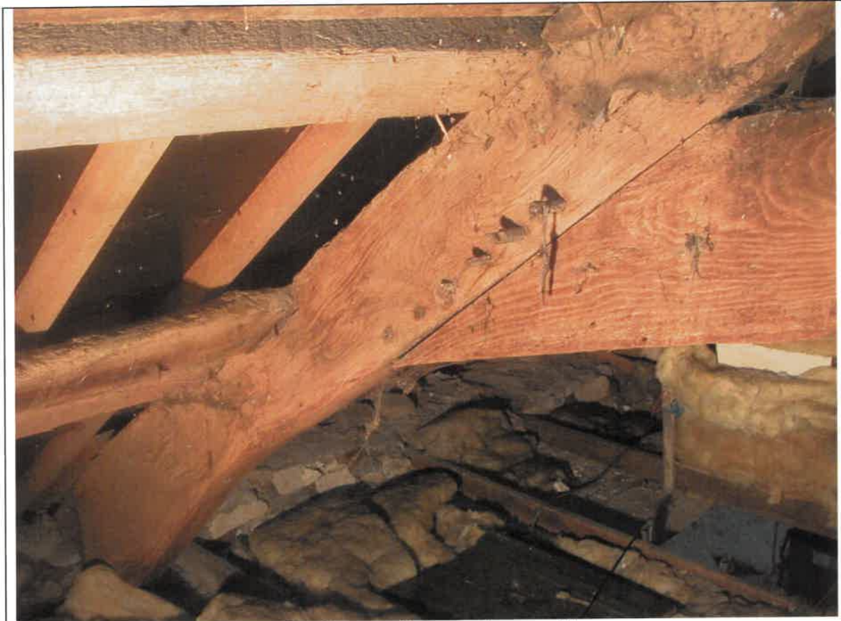
Plate 3 Truss 1 (viewed from south)
