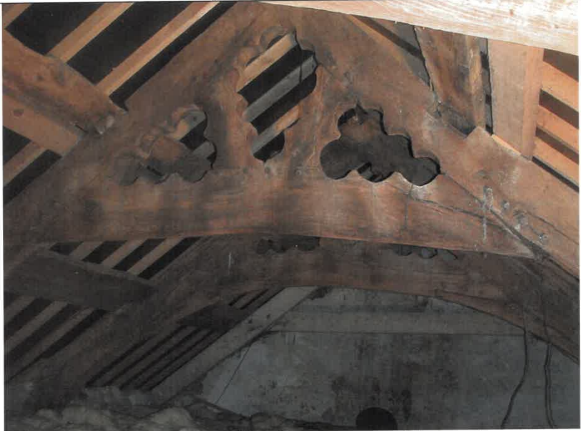
Plate 5 Trusses 2 & 3 (viewed from north - Truss 2 in foreground)
