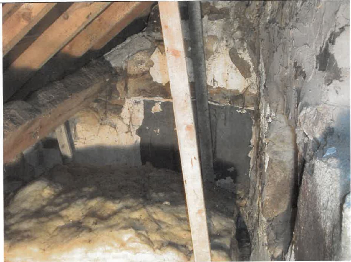
Plate 12 Possible blocked window in north gable
