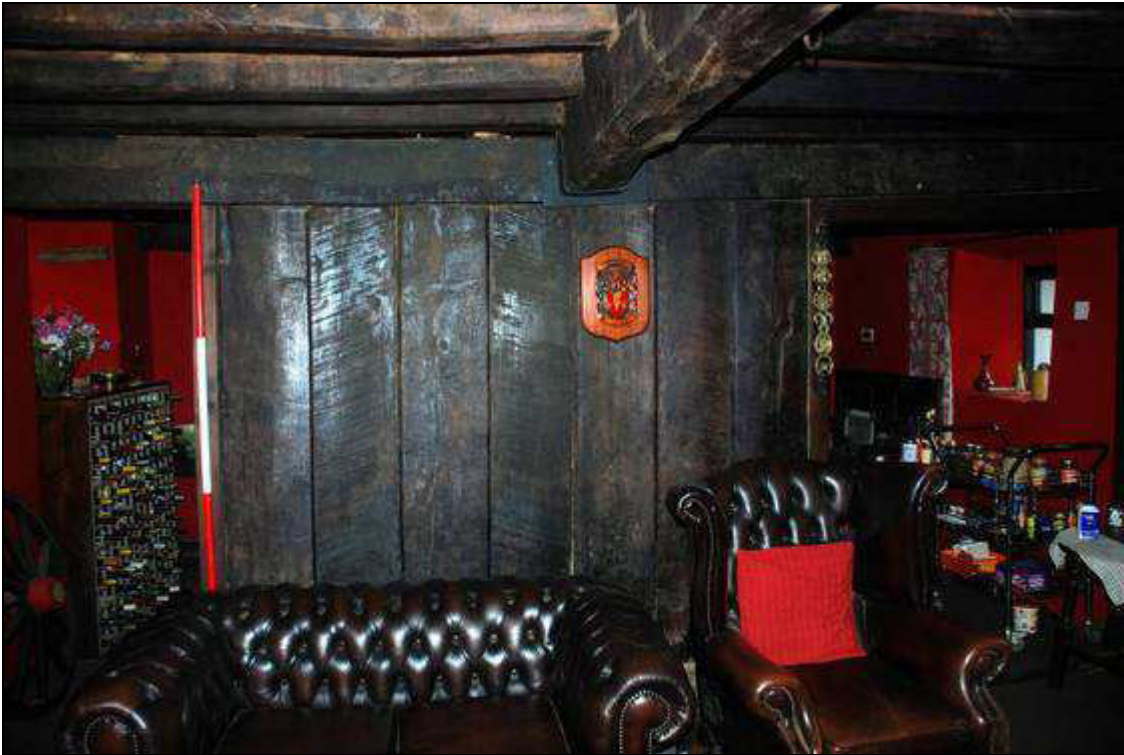
Plate 15: Post and Plank Partition looking south west
