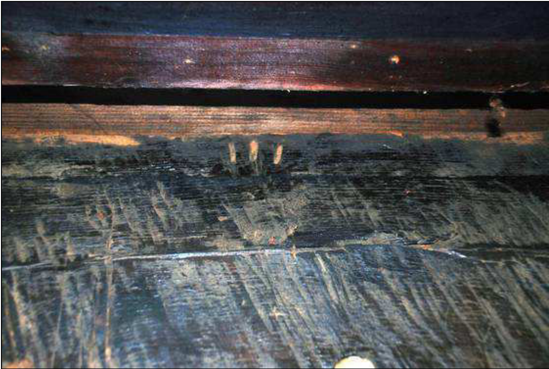
Plate 17: Carpenter's mark of "III" on partition
