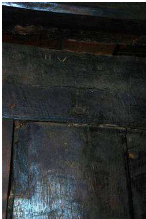
Plate 20: Carpenter's mark for "VII" on partition rail and post
