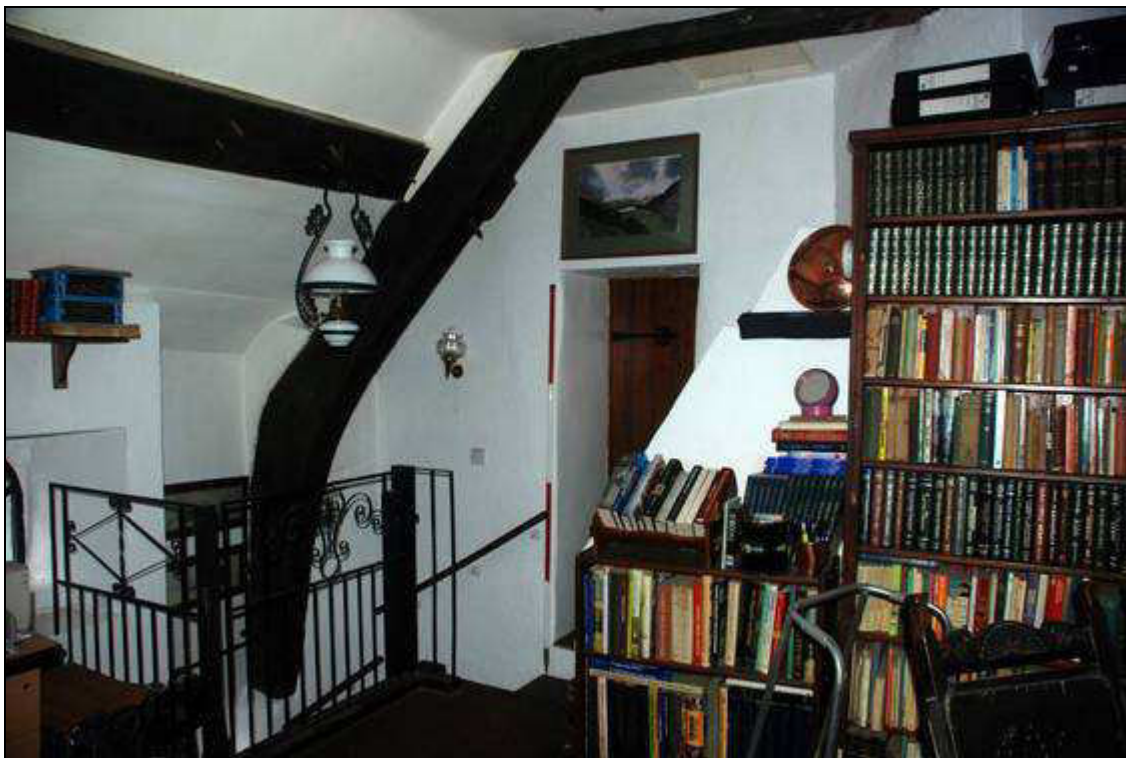
Plate 6: Truss 1, looking north
