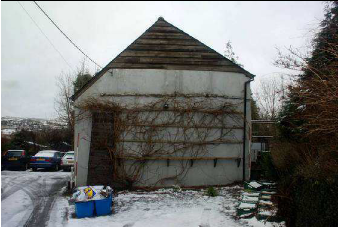
Plate 3: South west gable end
