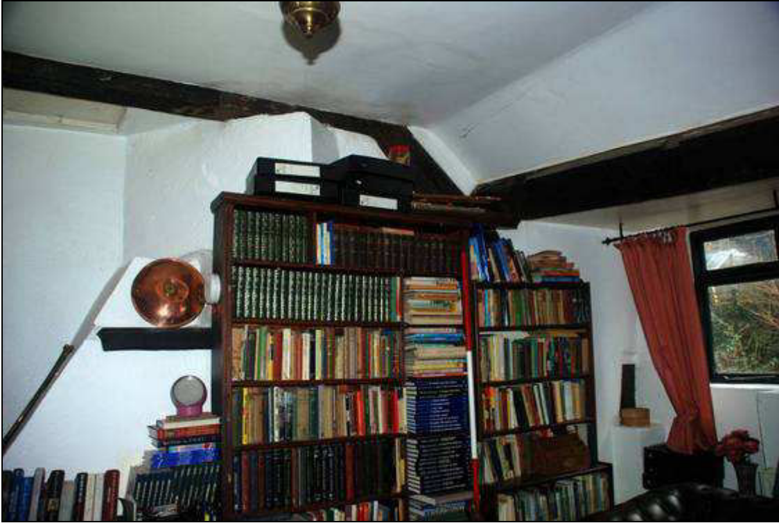
Plate 7: Truss 1, looking east
