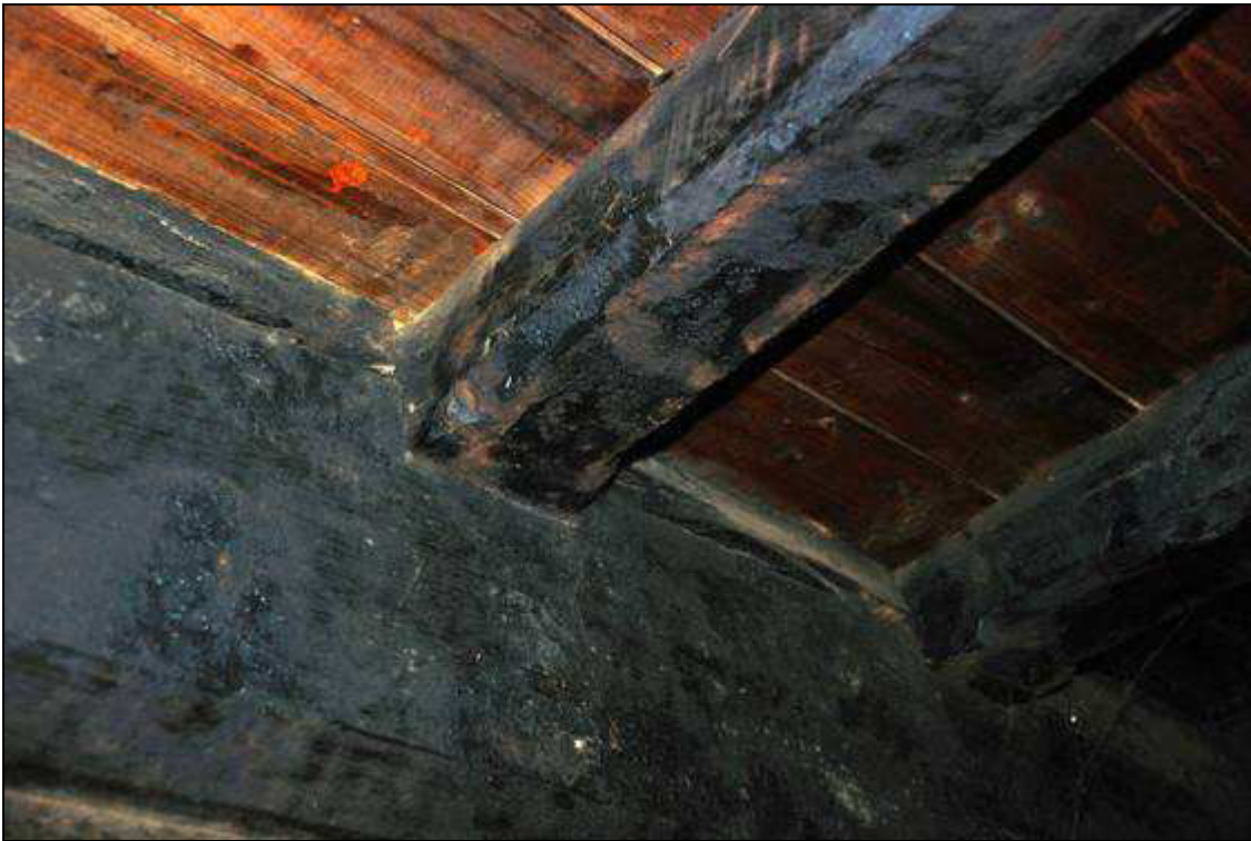
Plate 22: Joist in lower NE room, looking north
