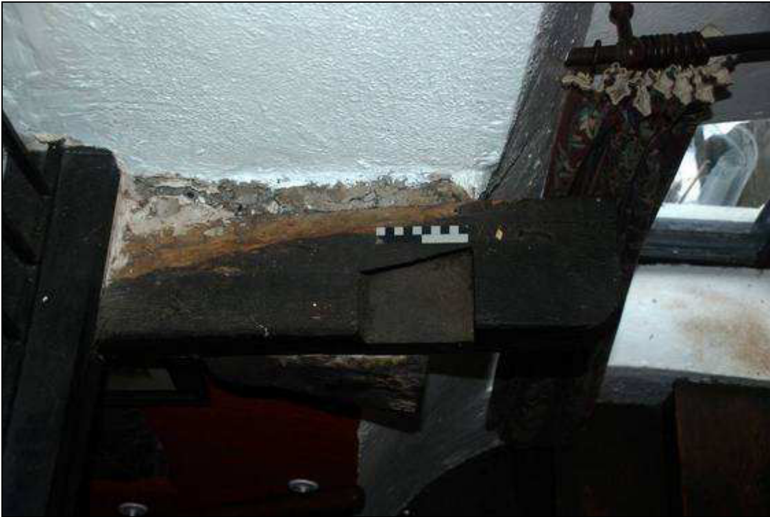
Plate 25: Rail truncated by the insertion of the stair case, looking down
