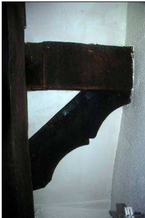
Plate 8: Windbrace and trussed joint on purlin
