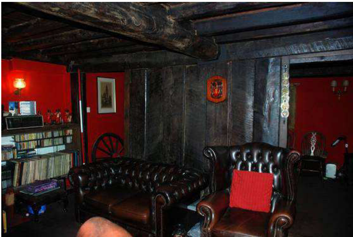
Plate 14: Post and plank partition looking south
