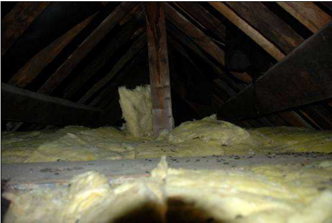
Plate 10: The roof space looking south west
