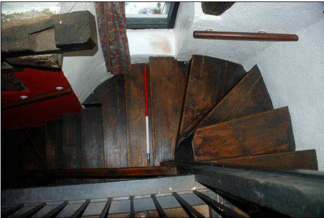
Plate 26: Curved recess in the staircase, looking down
