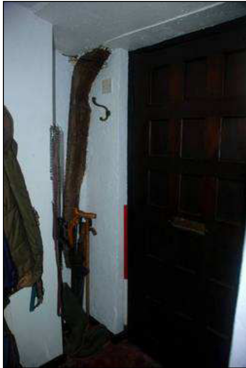
Plate 27: Re-sited door timber, looking west
