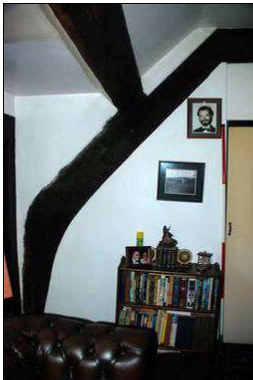
Plate 12: Truss 2, south east cruck, looking north
