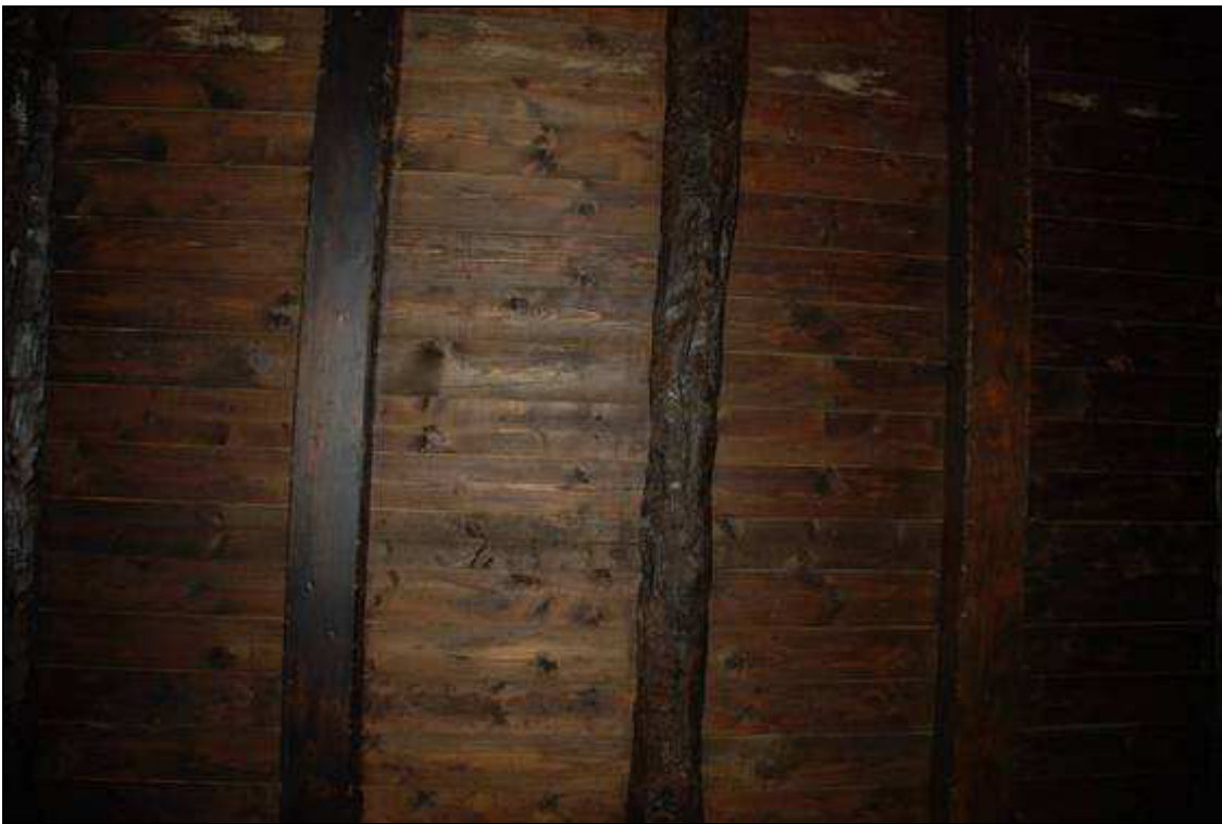
Plate 24: Variation between the ceiling joists in the SW ground floor room
