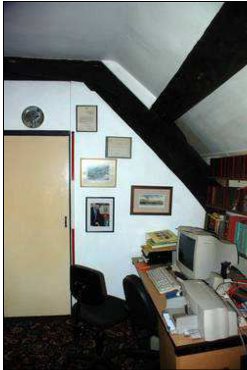
Plate 13: Truss 2, north west cruck looking west
