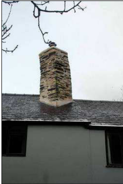
Plate 5: Chimney looking north west
