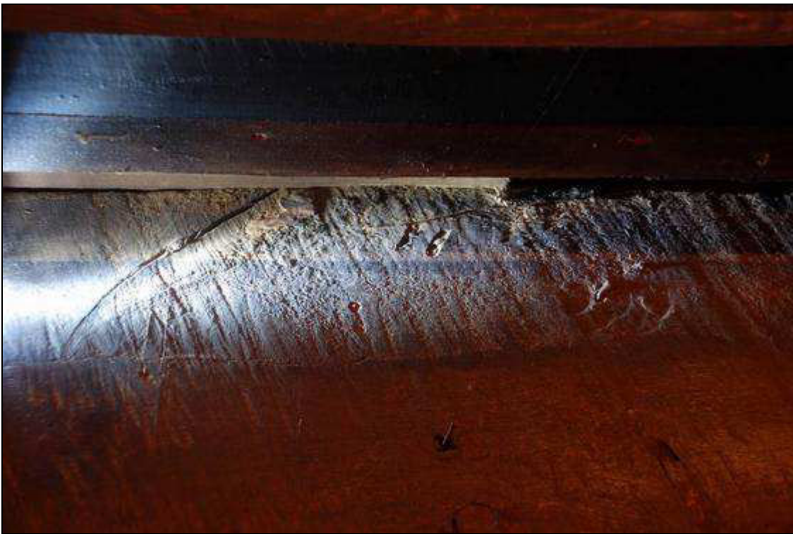
Plate 16: Carpenter's mark of "II" on partition
