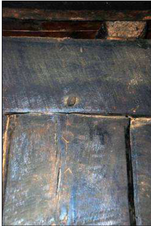
Plate 19: Carpenter's mark for "VI" on partition rail and post
