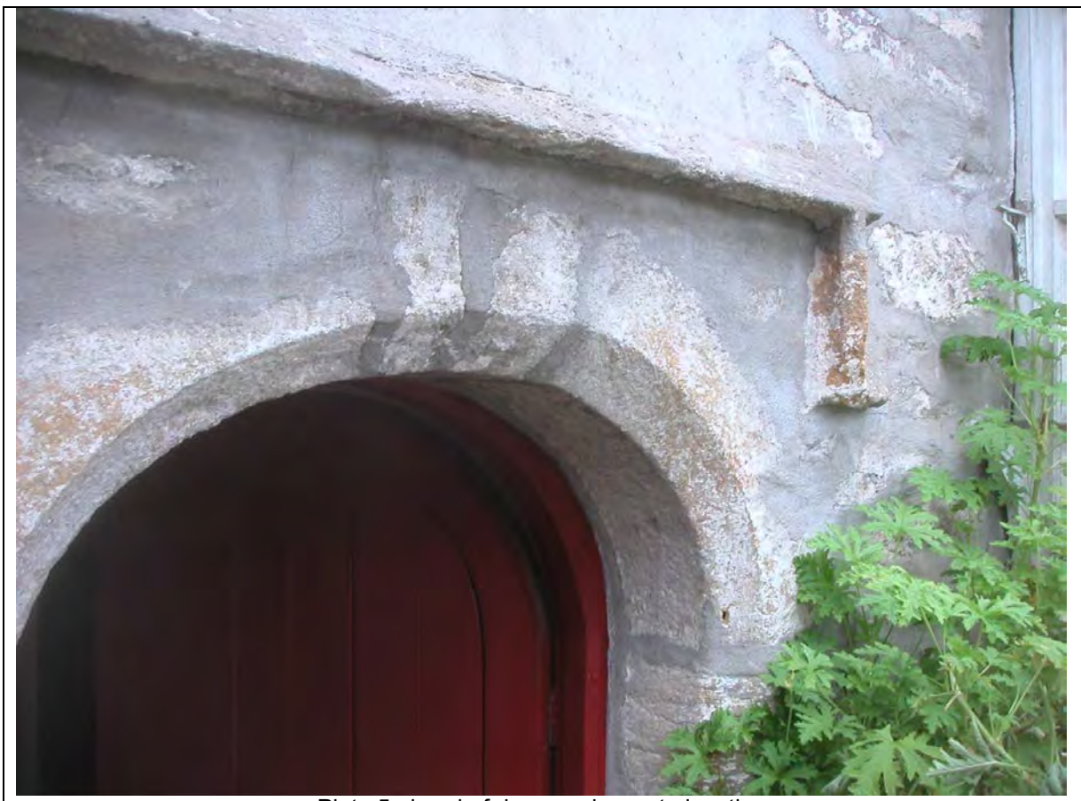
Plate 5 head of doorway in west elevation
