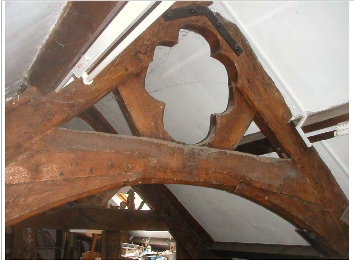
Plate 1 Truss 3, from south
