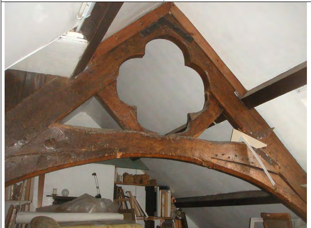
Plate 2 Truss 1, from south
