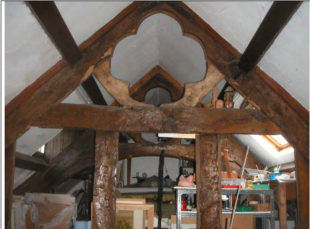
Plate 3 Truss 2, from south (truss 1 beyond)
