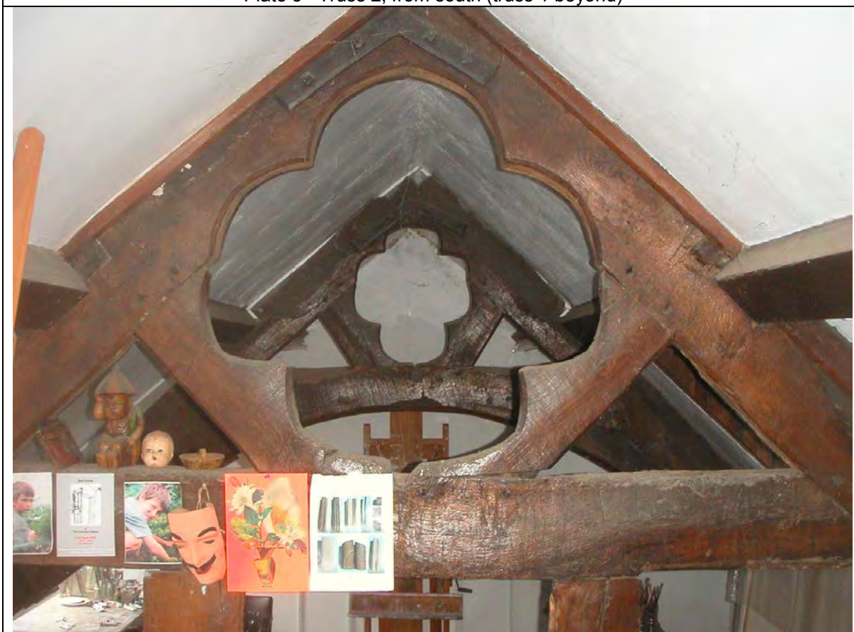
Plate 4 Trusses 2 & 3, from north
