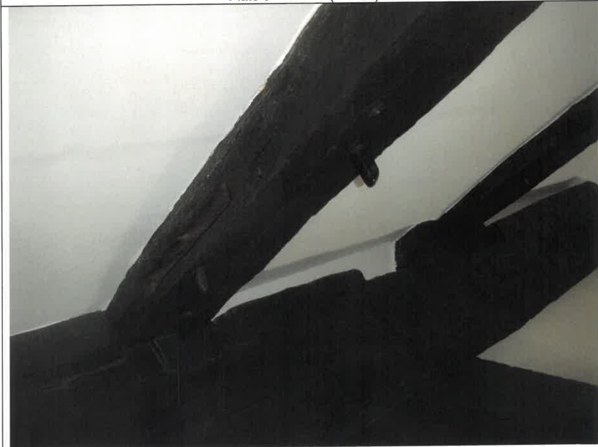
Plate 4 Truss 2 (slots and cut-outs for wind-braces)
