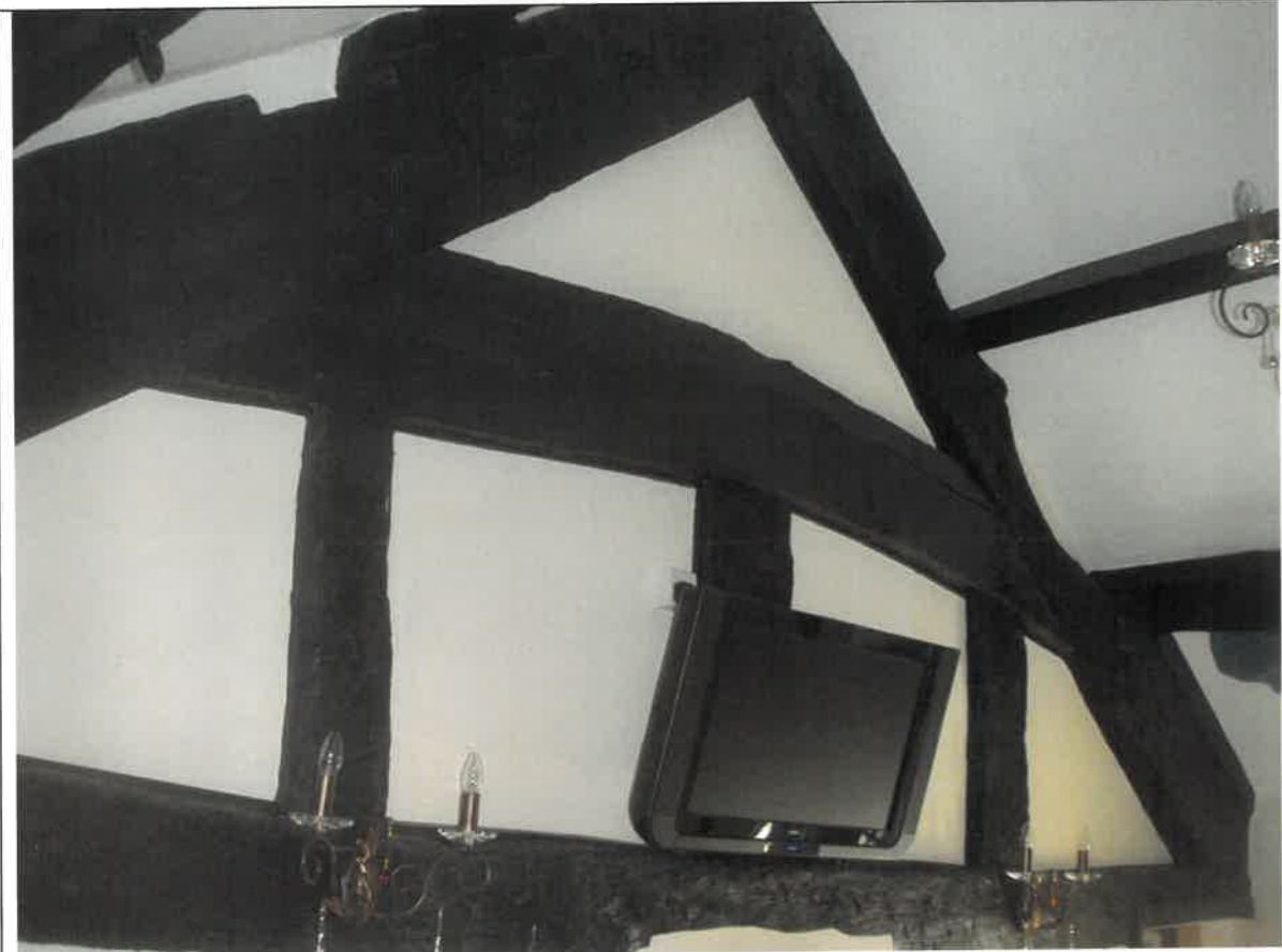
Plate 3 Truss 2 (W face)
