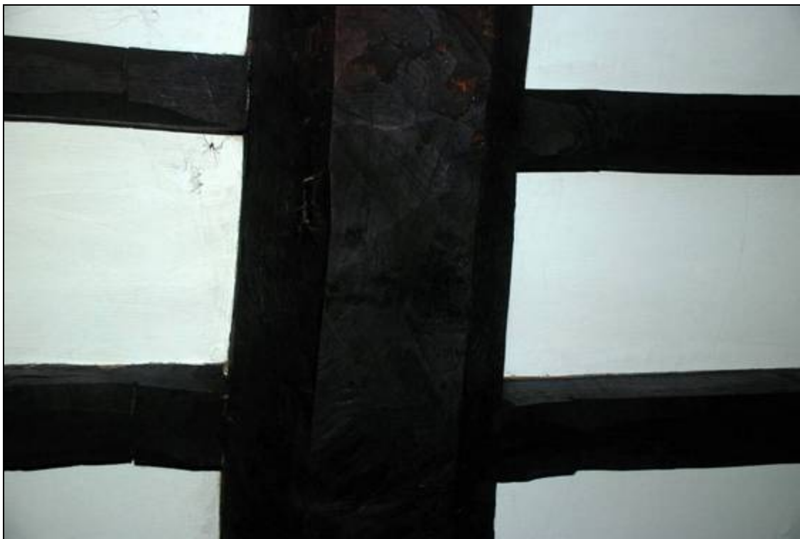
Plate 16: Chamfer and stops on the joists in the main room, looking up
