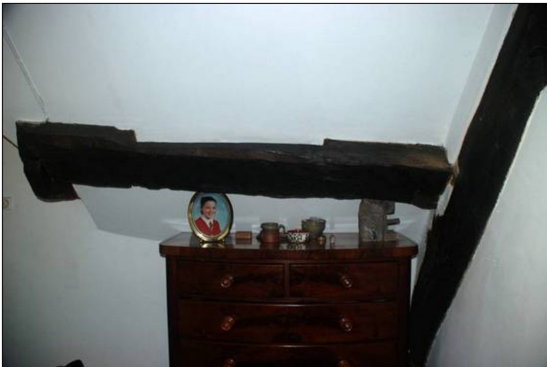
Plate 12: Lower purlin adjacent to Truss 3, looking south.
