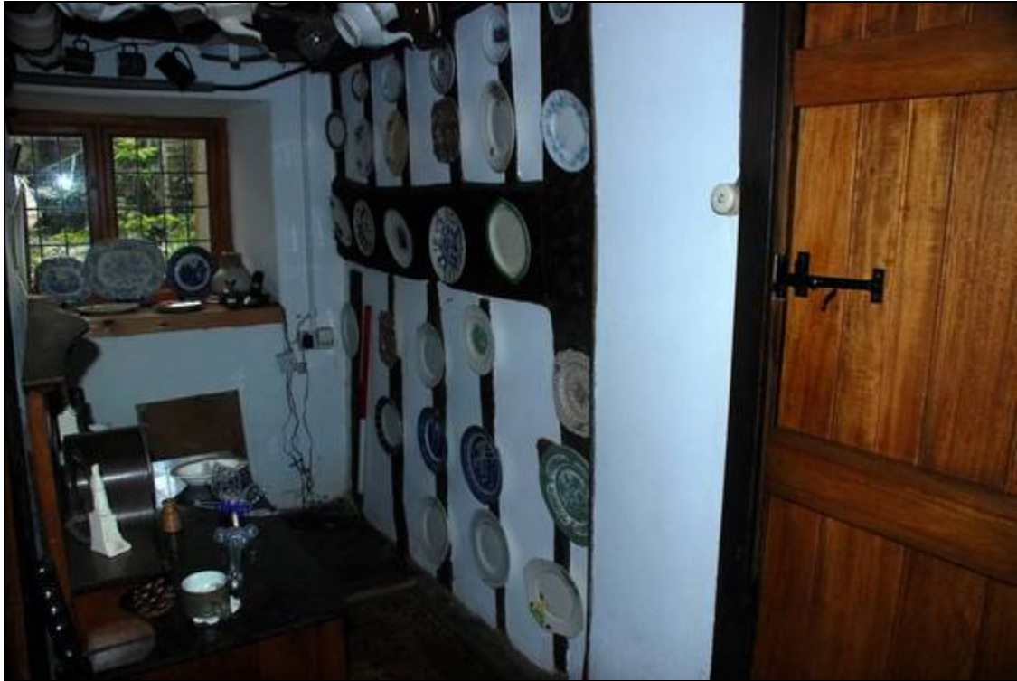
Plate 13: Stud and rail partition between the hall and kitchen, looking SW.
