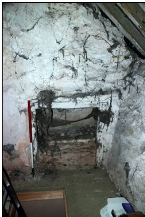
Plate 10: Blocked opening in western gable end, looking east.
