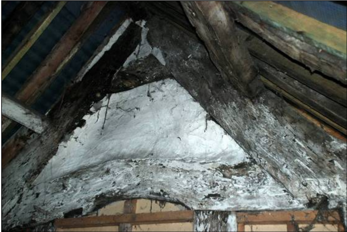
Plate 7: Lime plaster panel in Truss 1, looking west
