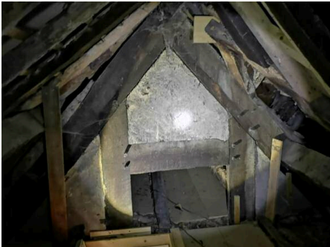
Fig. 6 - Wing partition framing in attic.
