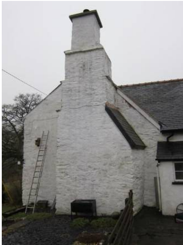
Fig. 7 - The external stone stack added to the parlour wing that was otherwise rebuilt within the footprint of the original cruck-framed hall house.
