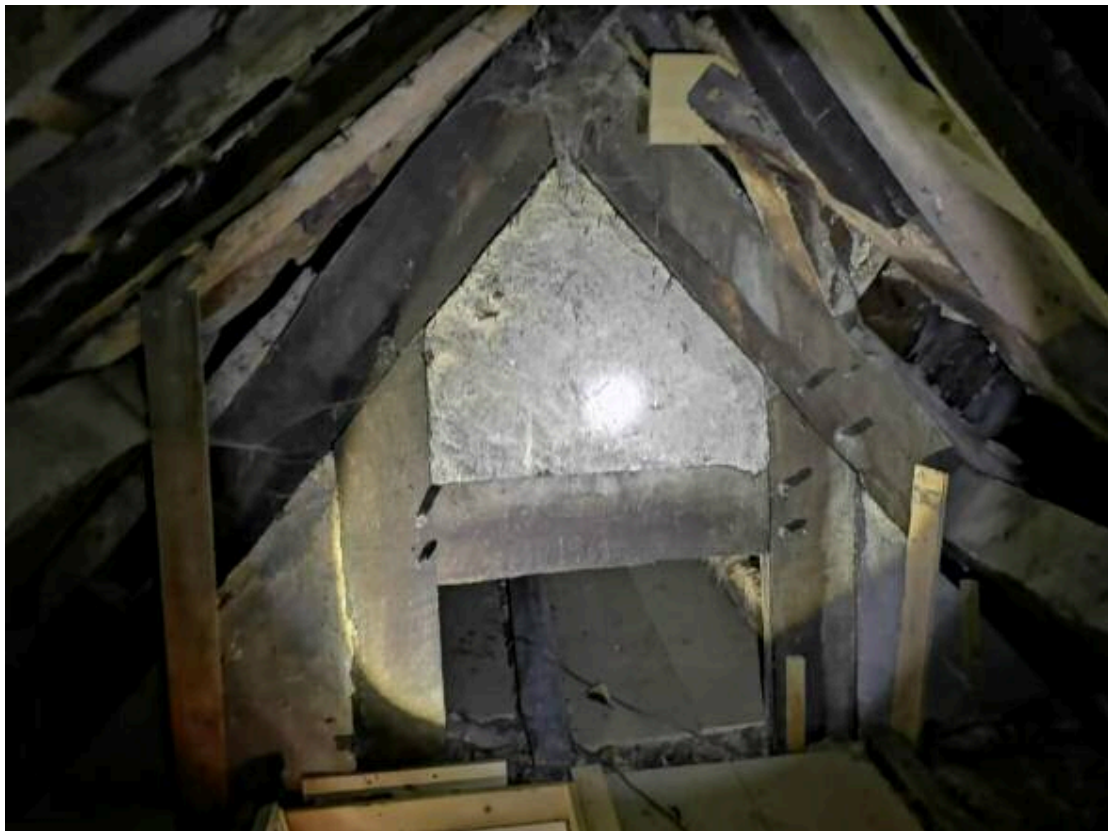
Fig. 6 - Wing partition framing in attic.
