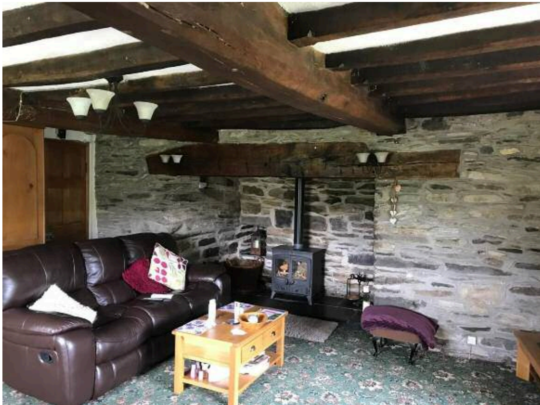
Fig. 4 – Parlour wing: ground-floor room, reconstructed after a fire, with slip tenoned joists. The chambers above this room were retained along with the principal rafter roof structure.
