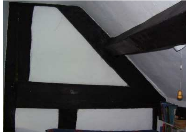
Fig 7. Part of cruck beam in upstairs bedroom.
