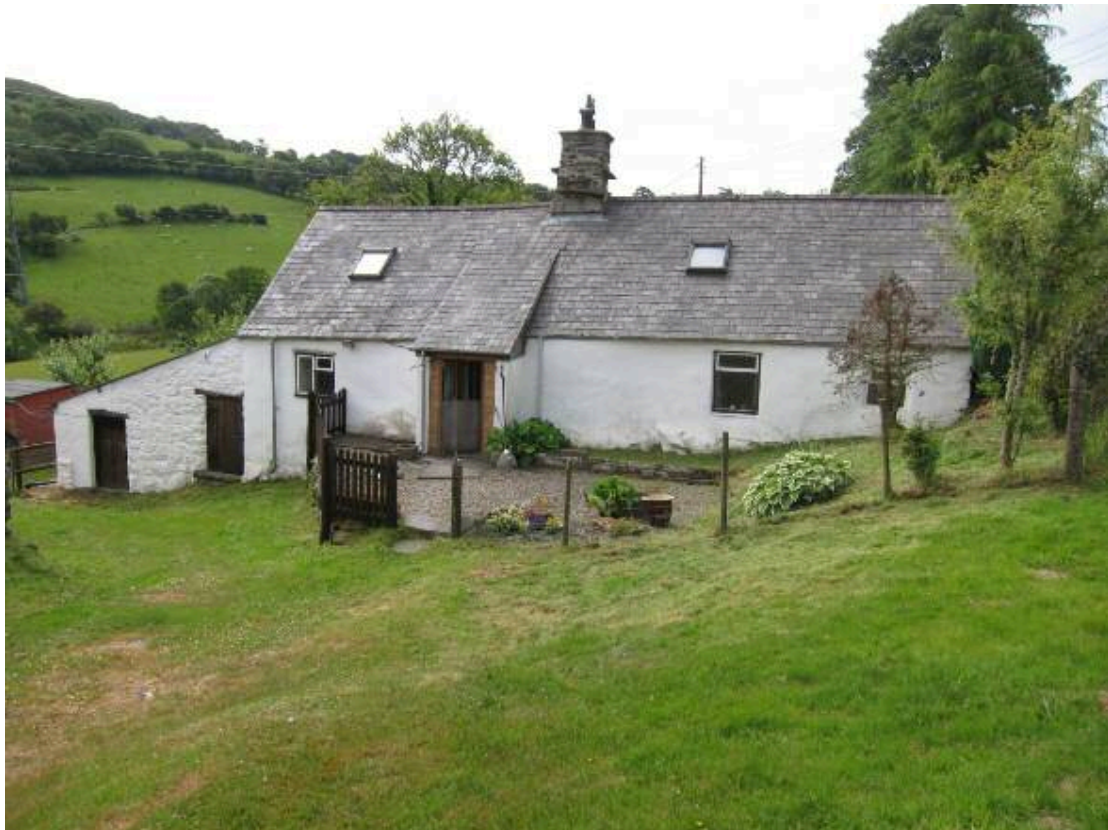
Rhydywernen, Llanfor from the north. The later porch marks the entrance to the former cross passage, incorporated into one of the bays of the open hall. The inner rooms are to the right.
