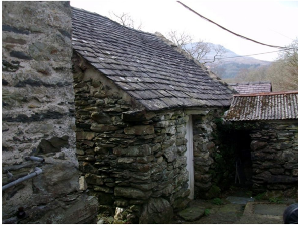
The dated outbuilding (above) in context (marked by arrow, right).
