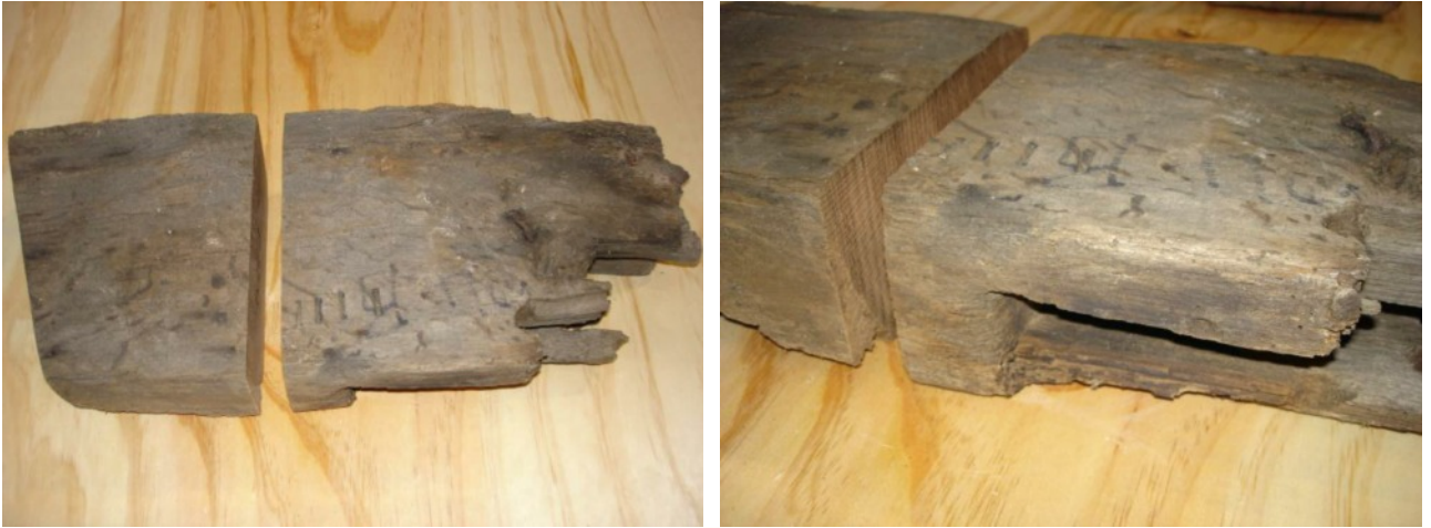
Fig 1c: Timber angg03 showing location of sample slice
