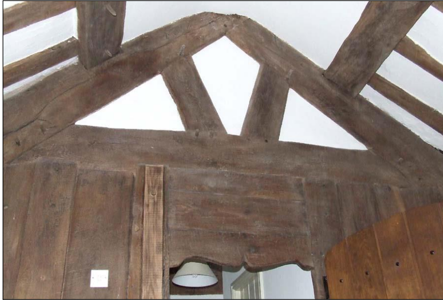
Figure 2: Plank and muntin panel on the first floor, thought to have been moved from the ground floor, with an inserted ogee doorhead.
