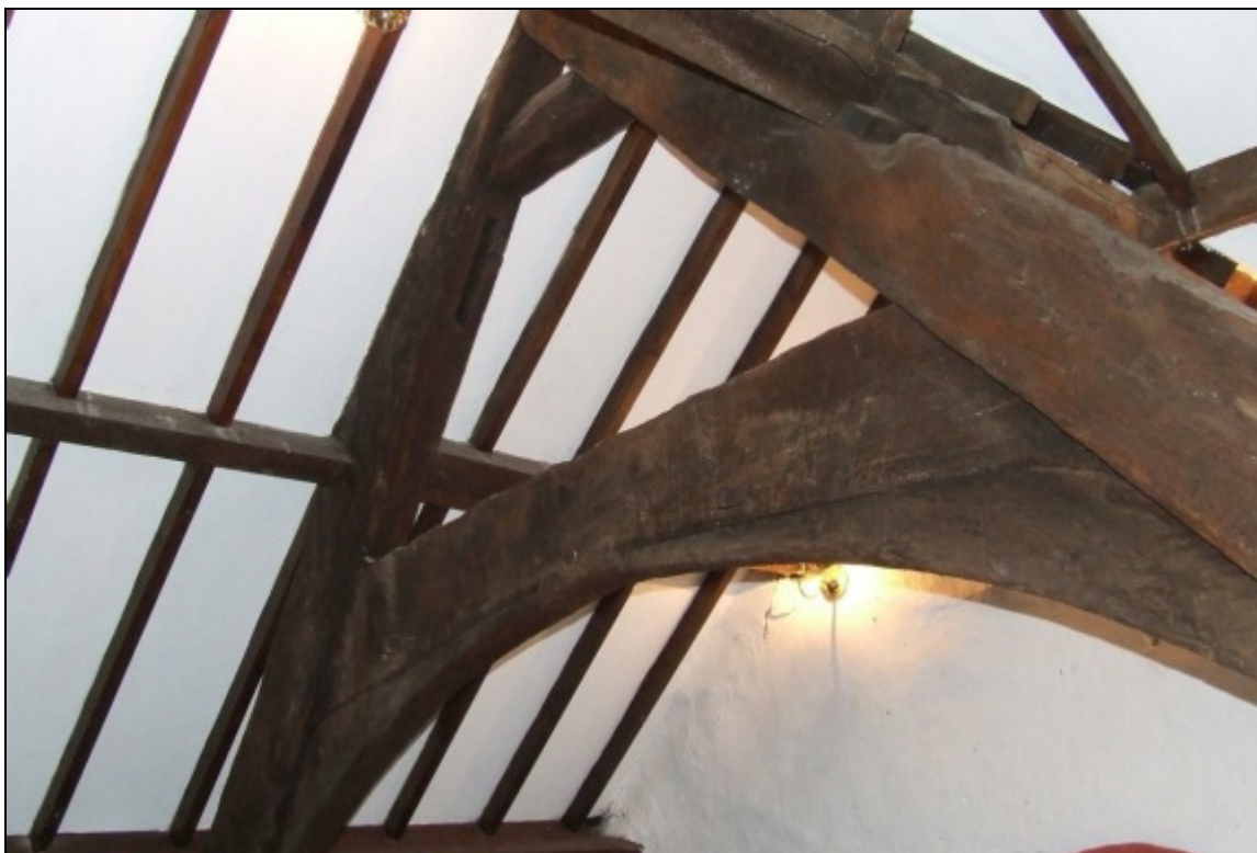
Figure 1: Cruck-truss at Cynfal Fawr.
