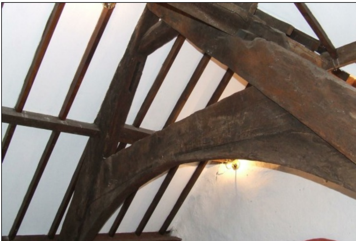
Figure 1: Cruck-truss at Cynfal Fawr.
